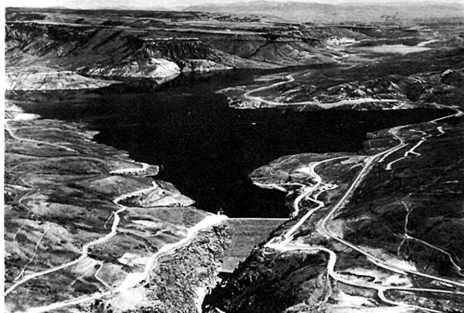
BLUE MESA DAM AND RESERVOIR
