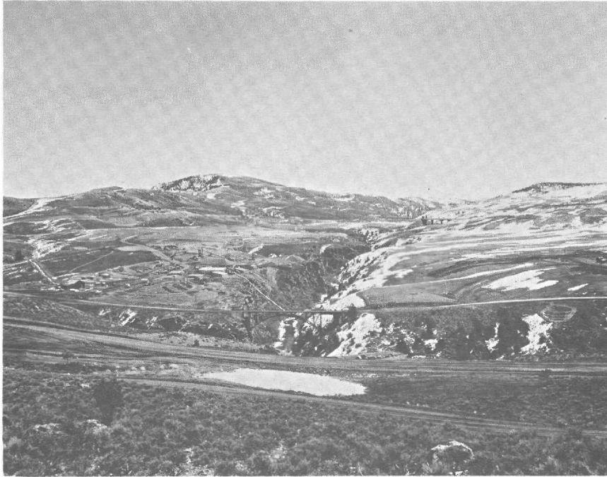
Blue Mesa reservoir site – view southeast up Lake Fork of Gunnison River. Bridge is on abandoned Highway 50 to be inundated; relocated highway in distance.
