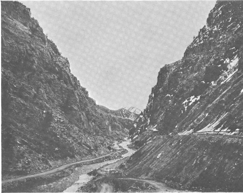
Morrow Point reservoir site – view up Black Canyon of the Gunnison River to damsite.
