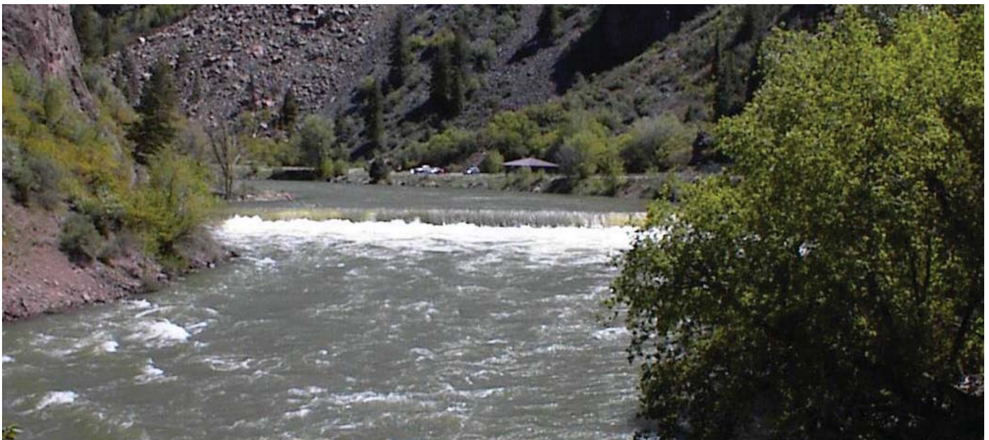
The Gunnison Diversion Dam at East Portal within Curecanti National Recreation Area, a feature of Reclamation’s Uncompahgre Project.
