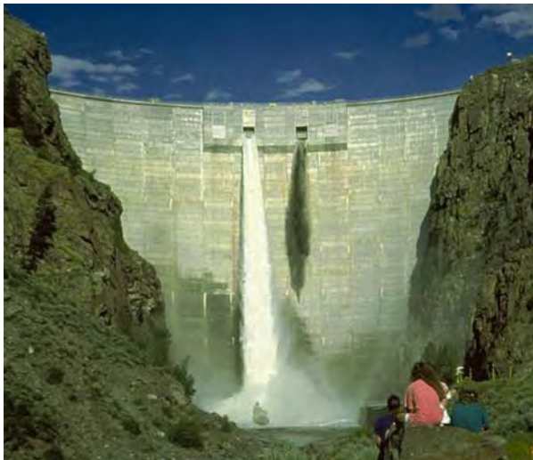
Morrow Point Dam, one of three large dams managed by Bureau of Reclamation within the Aspinall Unit at Curecanti
