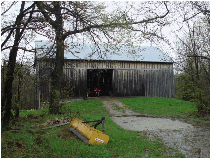
Earthen ramp to gain access to second floor of the bank barn (Jackson 2011)
