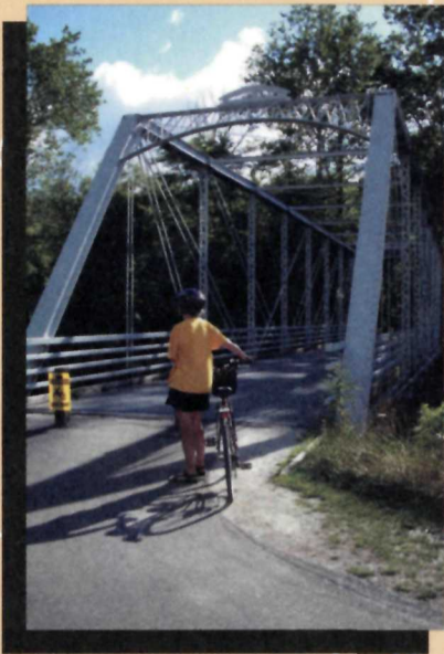
Station Road Bridge Area This section of the national park includes the narrowest part of the Cuyahoga Valley. The restored wrought-iron truss Station Road Bridge provides a link between hiking, equestrian, and all-purpose trails and the Towpath Trail.
