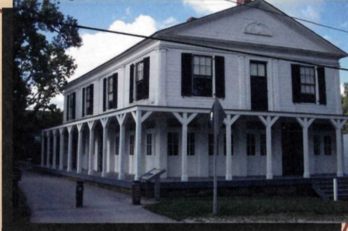
Boston Store This 1836 building, previously used as a warehouse, store, post office, and gathering place, is now a canal boat building museum featuring exhibits on all aspects of that business.
