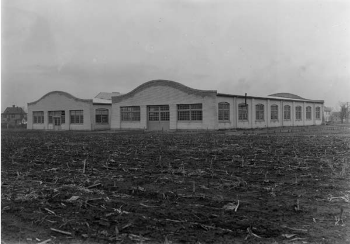
The Wright Company factory buildings, 1911. Image: Library of Congress, LC-DIG-ppprs-00712.
