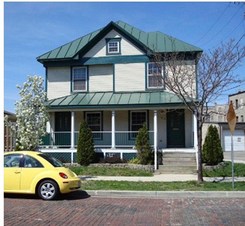
23 South Williams Street. (NPS 2007)
