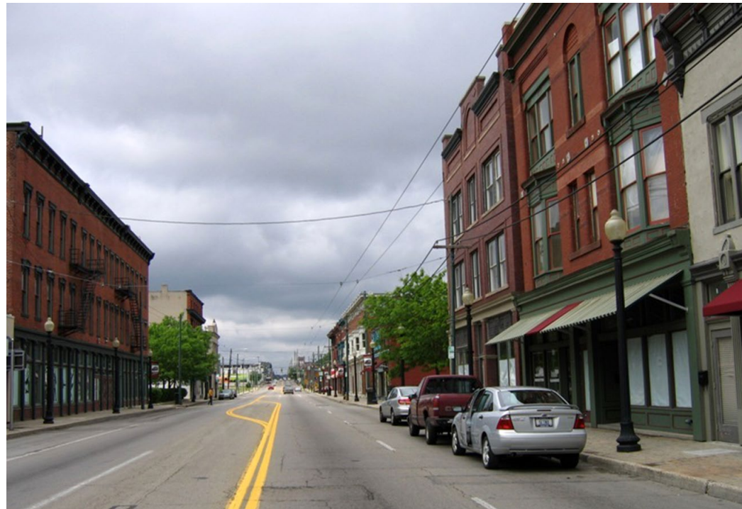
West Third Street, looking west. On the left, the Walters Block. On the right, from the right, the Gunkel Building (green awning) and the Webbert Flats. (NPS 2008)
