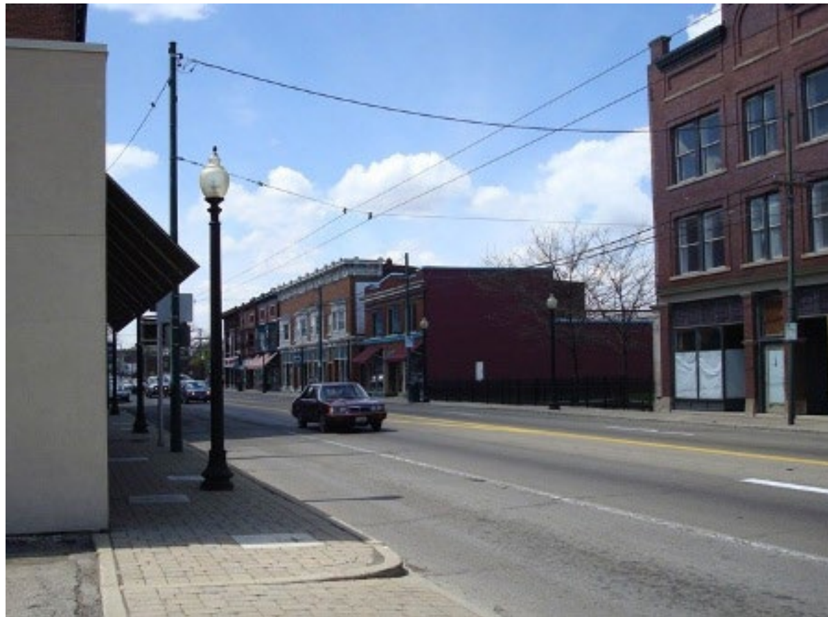
West Third Street, looking west. Starting from the right and moving left, the Webbert Flats (listed on the preceding page), the Hale Building (maroon awnings), and the Hoerstig-Holtman Building. (NPS 2008)
