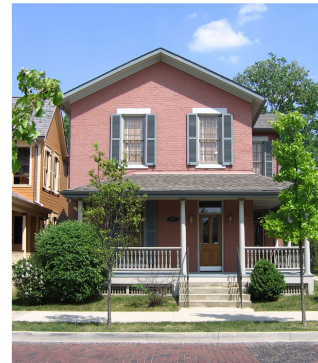
20 South Williams Street. (NPS 2007)
