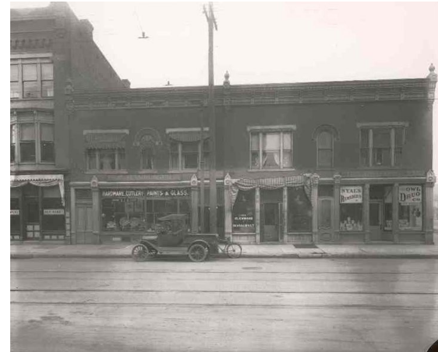
Gunkel Building, 1916. (Dayton Aviation Heritage National Historical Park Archives)
