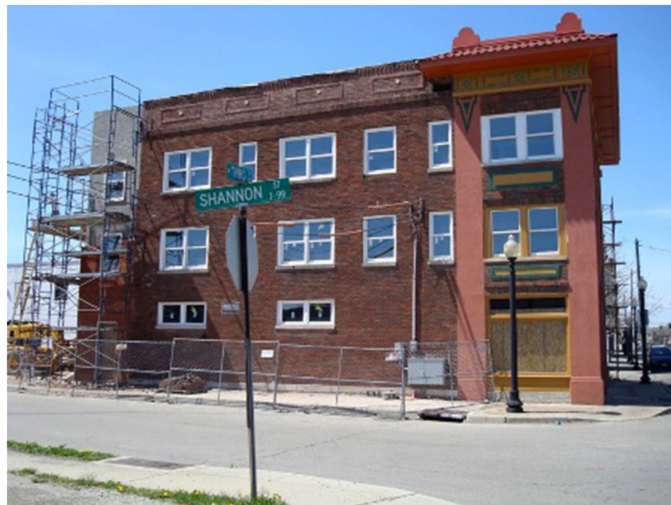
Allaman Building. (NPS 2008)
