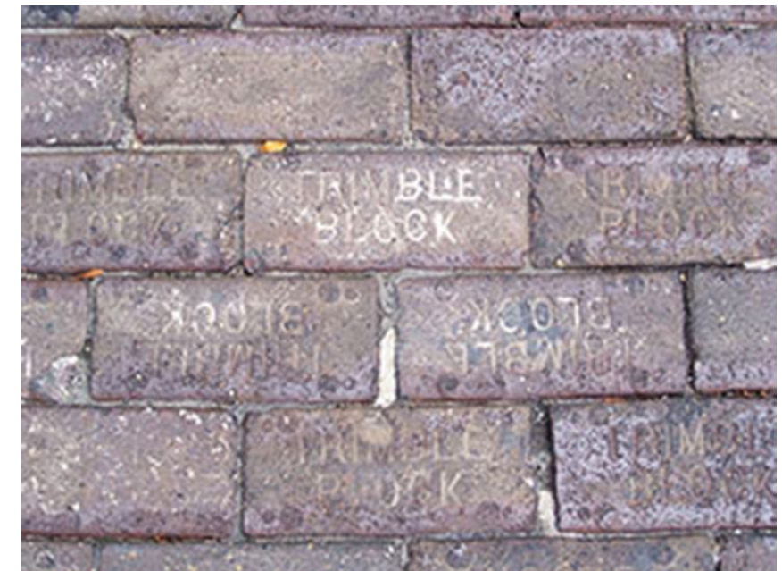
Detail of South Williams Street paving blocks, with TRIMBLE BLOCK embossed on the surface. (NPS 2013)
