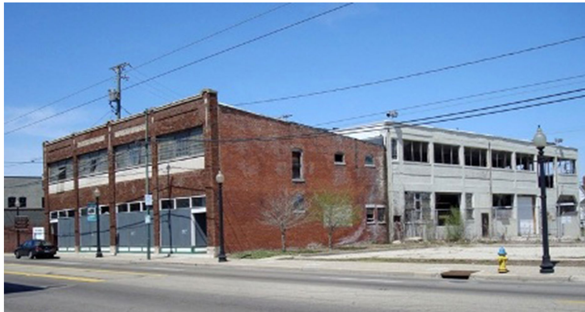
Gem City Ice Cream Building. (NPS 2008)
