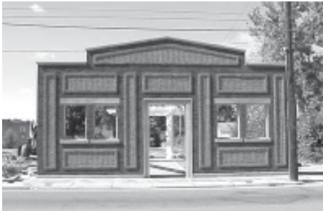
Facade of the Wright Engineering Laboratory, 15 North Broadway, October 2003.
