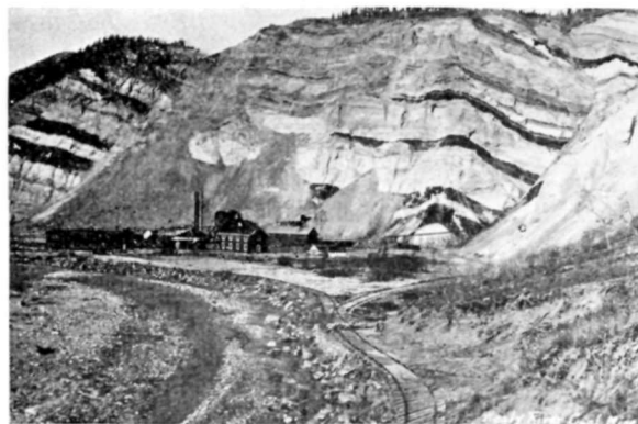
Sub Bituminous Coal Mine near Healy
