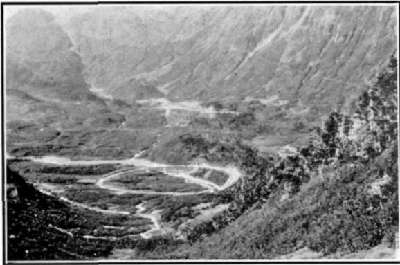
“Loop District” The Alaska Railroad
