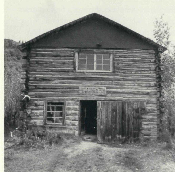
The Kantishna Roadhouse as it appeared in 1988
