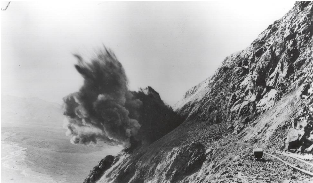
Blasting the High Line route (Alaska State Library, Alaska Road Commission Collection, 61-18-127).
