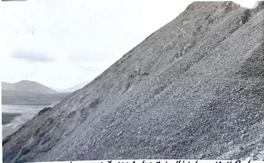
Foot trail on permanent road location. High Line, McK. P. July 1930
