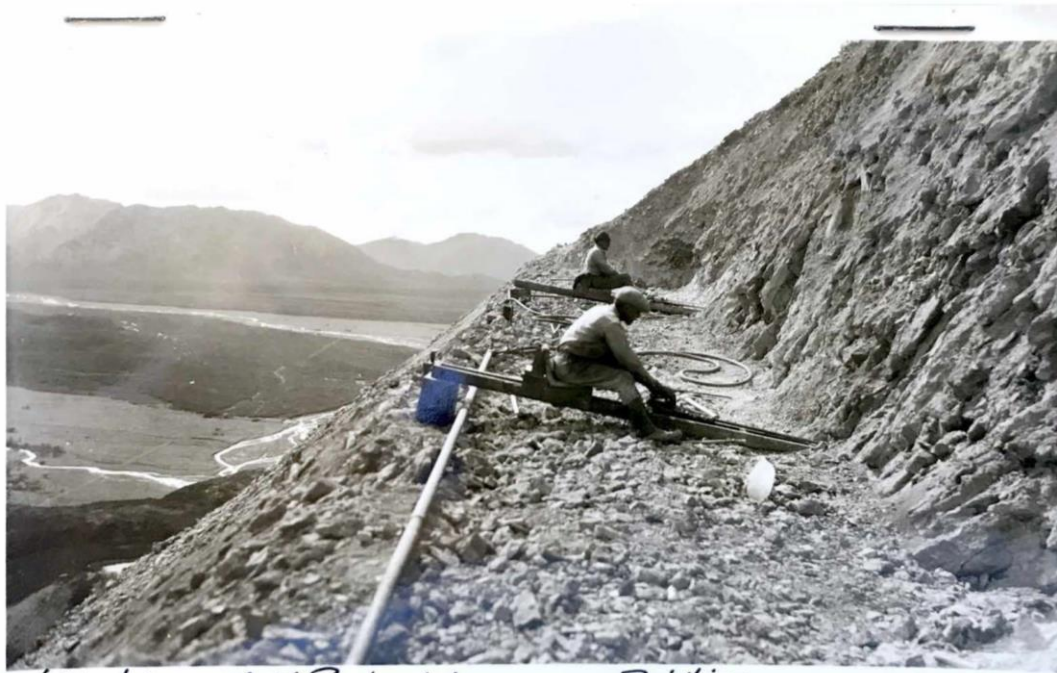
High Line, McK. Park, July, 1930. Drilling
