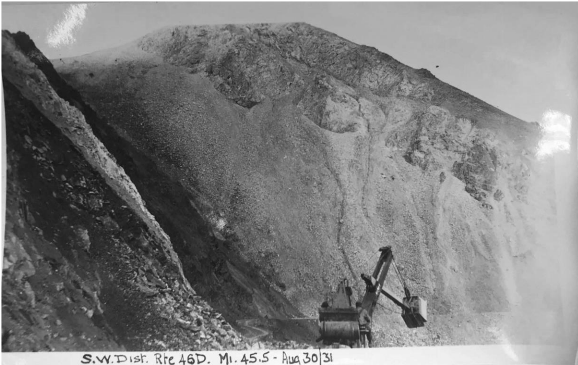
High Line Road being built in 1931 (Edmunds Collection, Box 1, Anchorage Museum)
