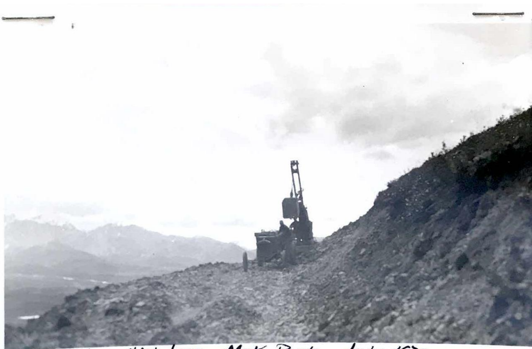
Grading High Line McK. Park July 1930
