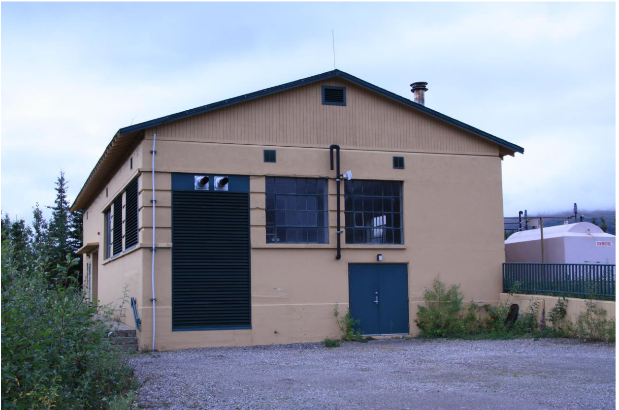
6 of 15. The Power House, north elevation, looking southeast (Photographer: Larissa Rudnicki, Date Photographed: August 16, 2011).
