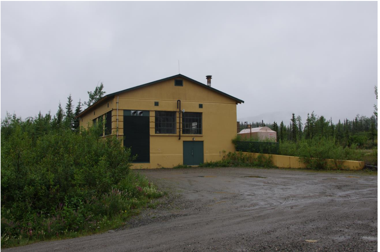
2 of 15. The Power House, overview, looking southeast at north elevation.
