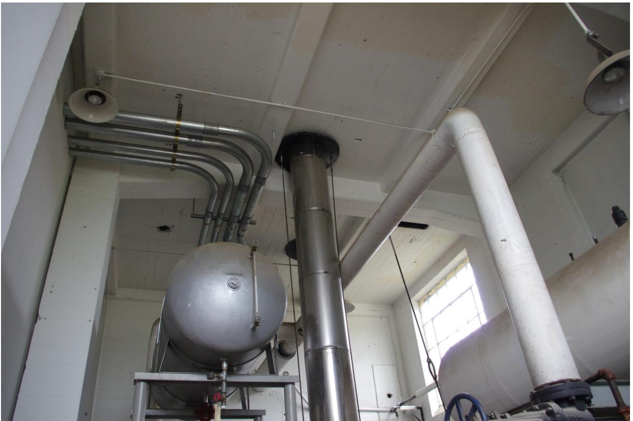
10 of 15. The Power House, interior, boiler room, looking southeast.
