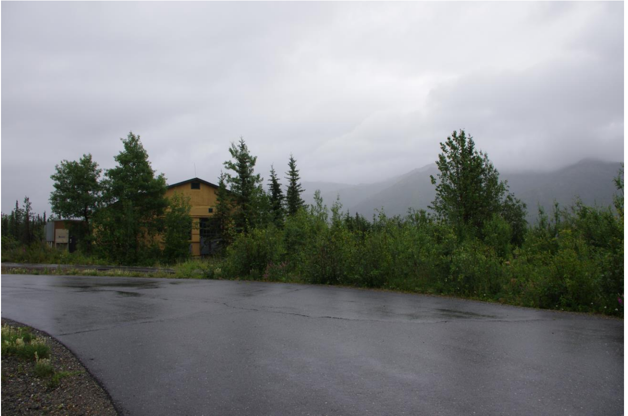
5 of 15. The Power House, overview, looking northwest at south elevation.
