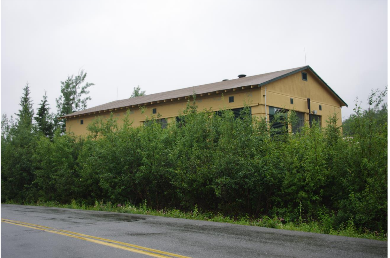
1 of 15. The Power House, overview, looking south toward east (facade) and north elevations.
