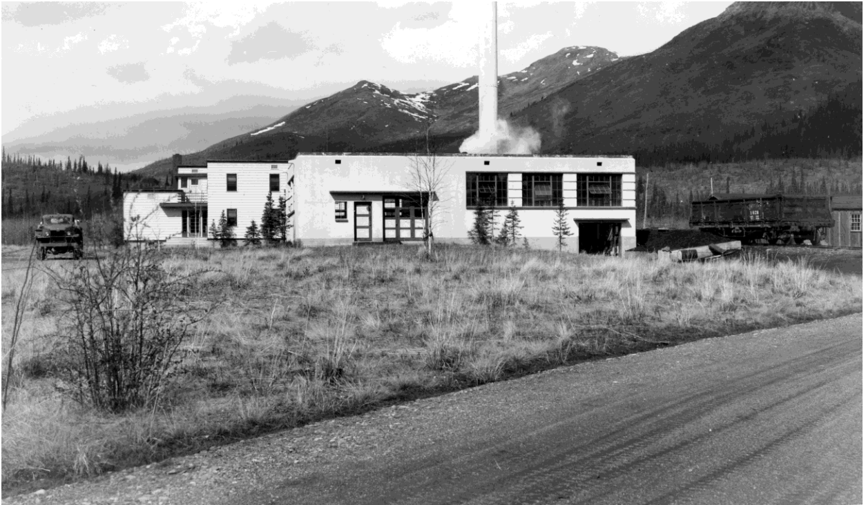
15 of 15. The Power House, “[Hotel powerhouse],” c1942-1943, unknown photographer, Catalog No. DENA-00532, Denali National Park and Preserve Museum Collection Archives, Denali National Park and Preserve, AK.
