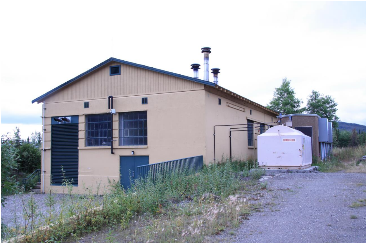
7 of 15. The Power House, north and west elevations, looking southeast (Photographer: Larissa Rudnicki, Date Photographed: August 16, 2011).
