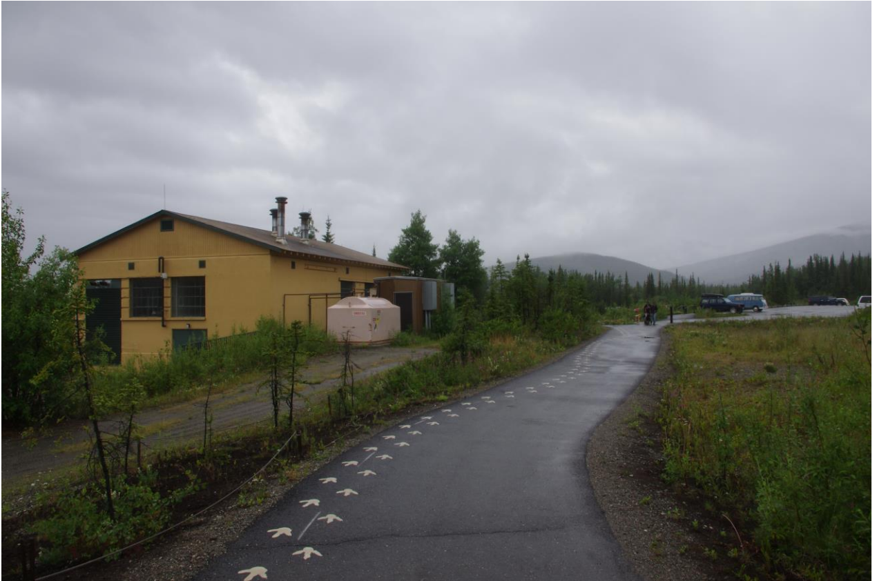
3 of 15. The Power House, overview, looking southeast at north and west elevations.
