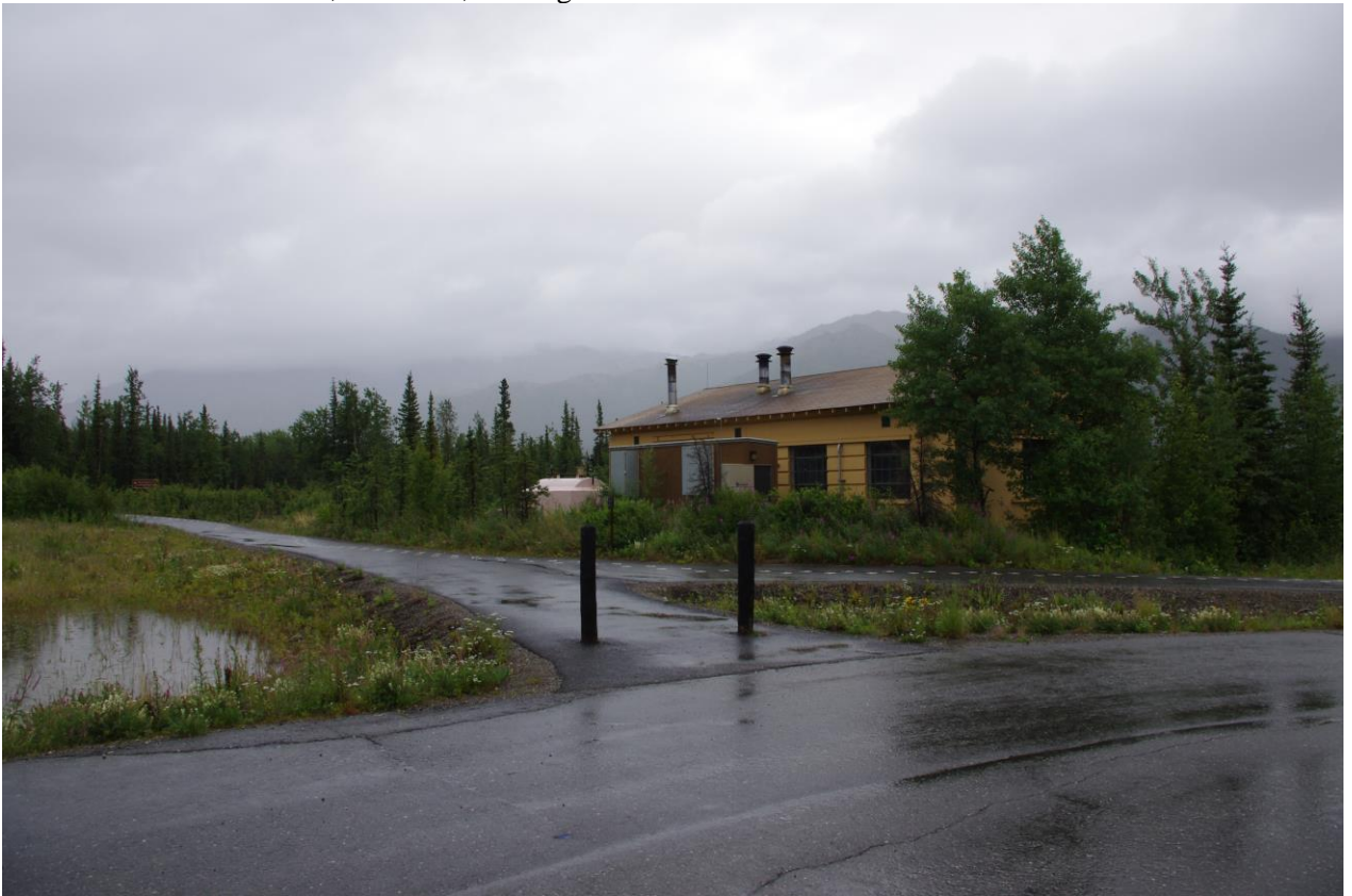
4 of 15. The Power House, overview, looking north at west elevation.
