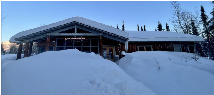
Figure 4. The Murie Science and Learning Center at Denali with heaps of snow on December 30, 2021. NPS Photo.
