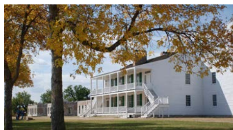
The restored Old Bedlam building at Fort Laramie National Historic Site NPS
