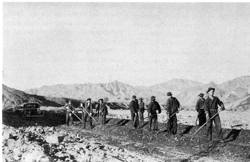
ROADS ARE EASILY BUILT AND SCARIFIED
