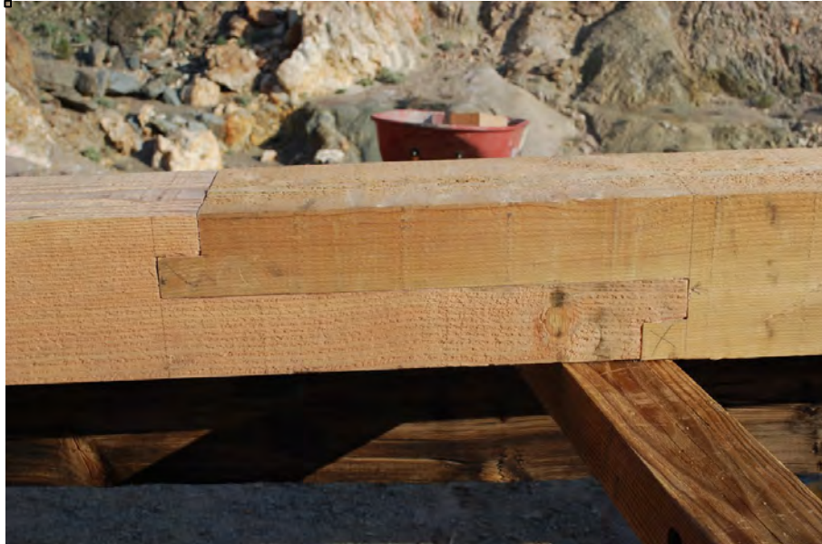
Figure 9. Bladed scarf joint splice for replacement column, tower 6.
