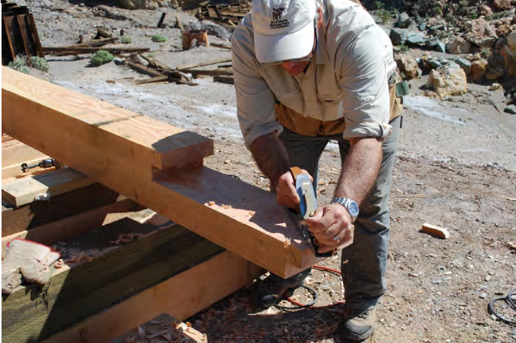
Figure 10. Planing face of scarf joint, replacement timber for tower 9
