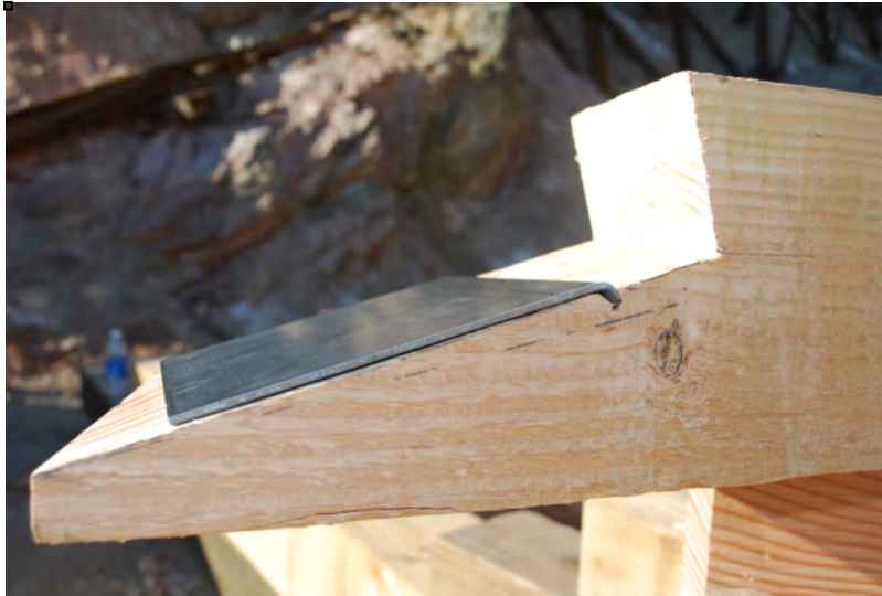
Figure 8. Replacement saddle beam brace with shear plate installed.
