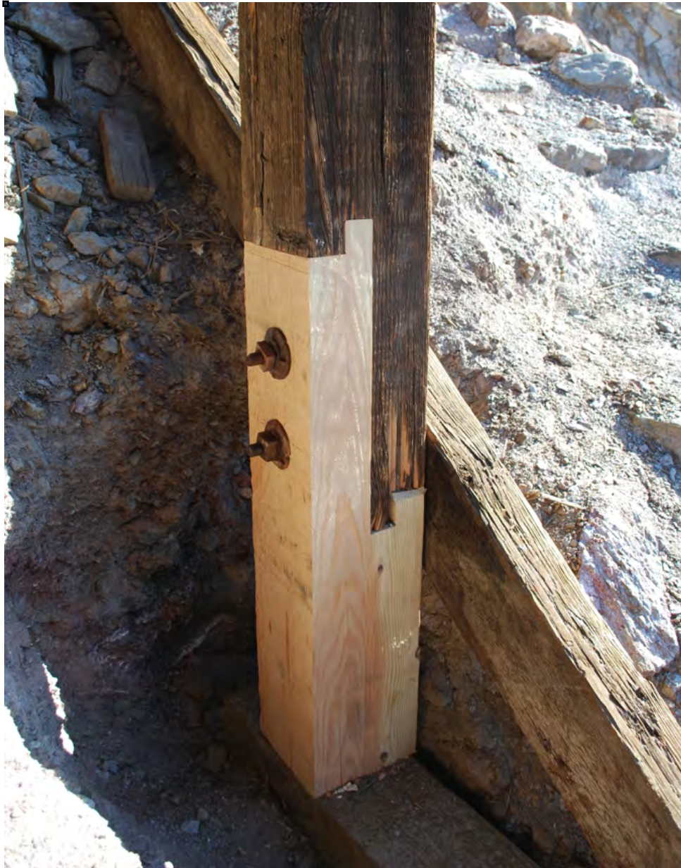
Figure 7. Column repair at A2, Lower Terminal.
