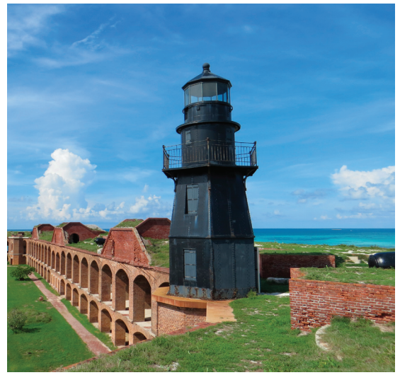
1876 Harbor Light Atop of Fort Jefferson
