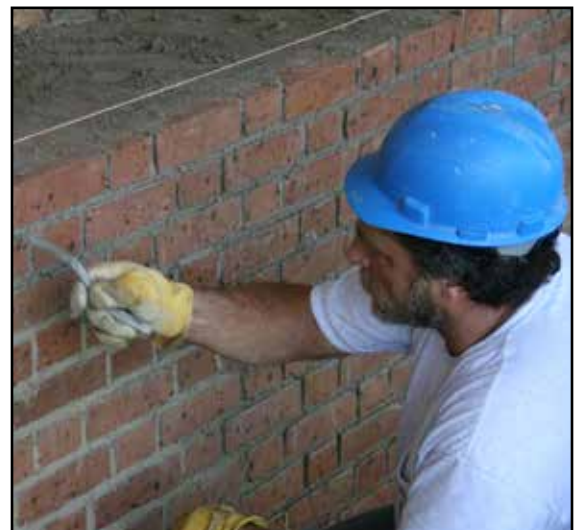
Masonry crew member tooling the joints
