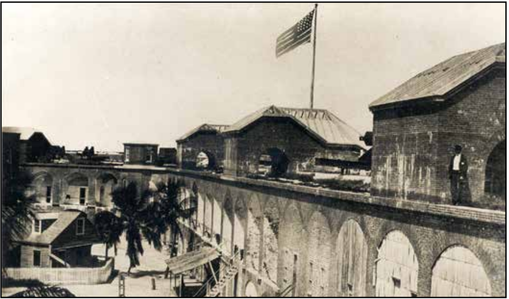
Front 3 with sallyport, below lean-to structure, lighthouse keepers house, and 2nd tier casemates converted to housing. (ca. late 1860s)
