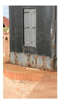
The condition and stability of the Harbor Lighthouse structure is likely to decline rapidly without immediate treatment. General maintenance and intermittent repairs performed in the 1930s, 1970s, 1990s, and 2000s have performed reasonably well and have allowed preservation of the structure for 140 years. However, continuing deterioration and shortening maintenance cycles indicate that the structure is on a downward course.
