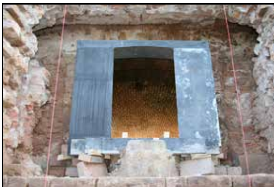
Replicated Totten Shutter components to be embedded within scarp wall
