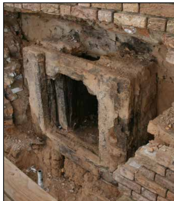
Original iron Totten Shutter assembly embedded within the scarp wall
