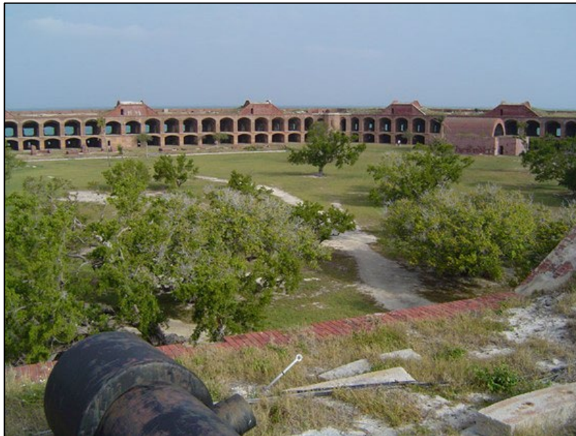
Fig 17. Parade ground looking north from terreplein, 2005.
