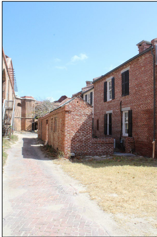
Fig 44. Brick walkway (April 20, 2022, photograph by Elizabeth Koreman).
