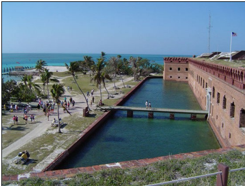
Fig 15. Moat and bridge, existing conditions, 2005.
