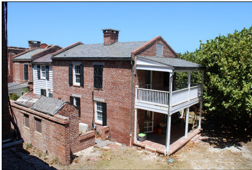
Fig 32. Staff House (Engineer's officers' quarters) (April 20, 2022, photograph by Elizabeth Koreman).
