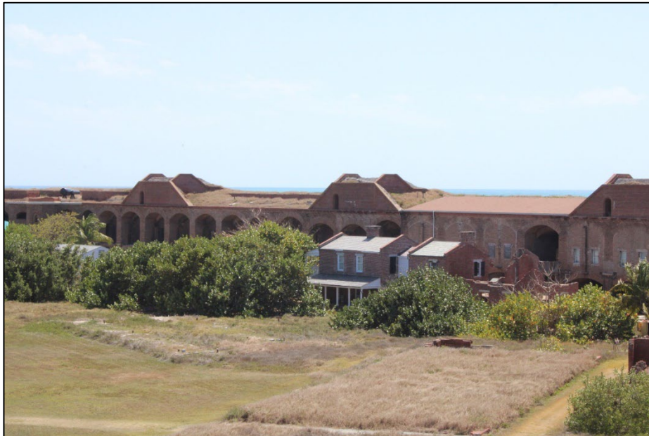
Fig 59. Leaching fields (April 20, 2022, photograph by Elizabeth Koreman).
