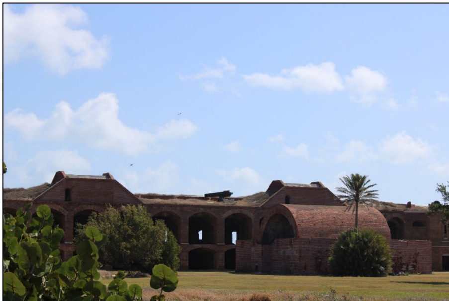
Fig 25. Large Magazine (April 20, 2022, photograph by Elizabeth Koreman).
