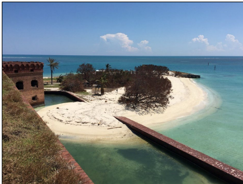
Fig 35. Moat filled with sand, post-Hurricane Irma (Photograph provided by Glenn Simpson, DRTO Park Manager).
