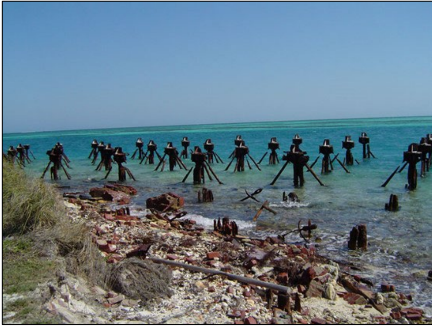
Fig 18. North coaling piers, 2005.
