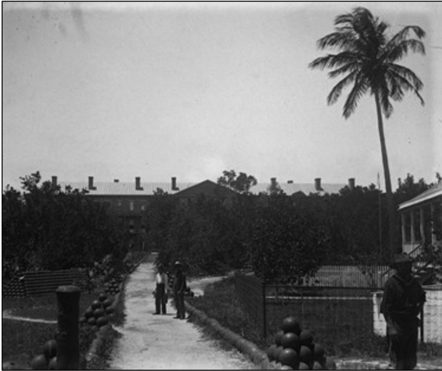
Fig 42. Walkway (c. 1909), Meigs collection, Number 54.
