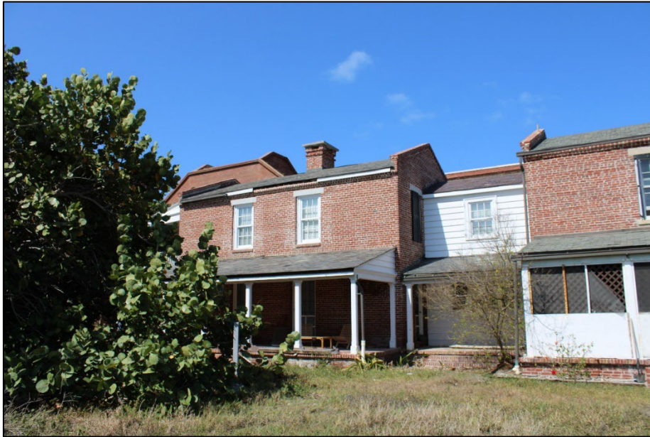
Fig 33. Staff House (Engineer's officers' quarters) (April 20, 2022, photograph by Elizabeth Koreman).
