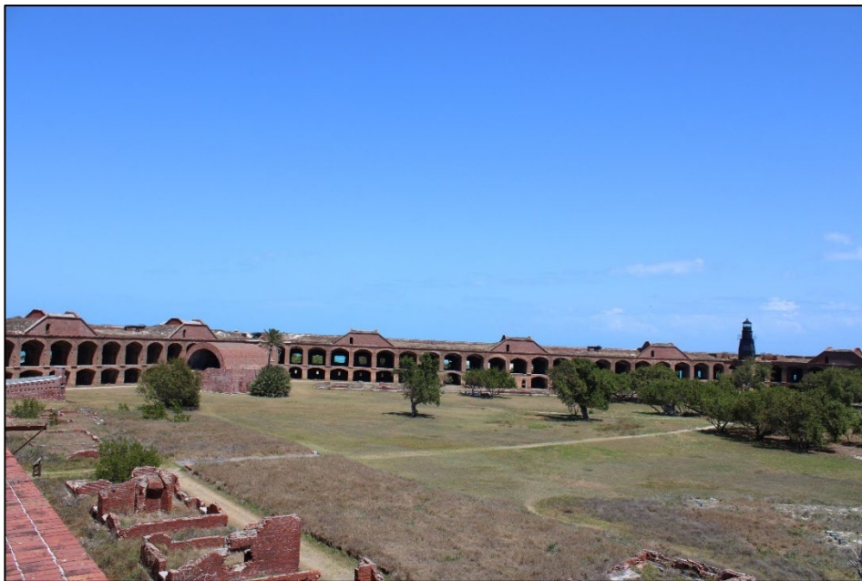
Fig 57. Parade ground (April 20, 2022, photograph by Elizabeth Koreman).
