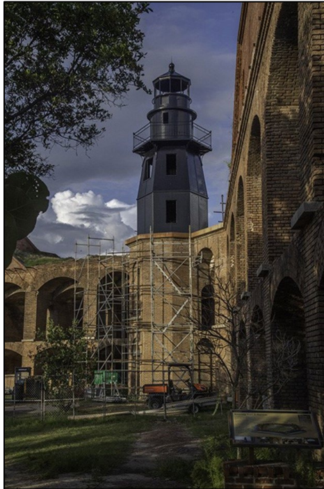
Fig 24. Harbor Light Restoration (Photograph provided by Glenn Simpson, DRTO Park Manager).
