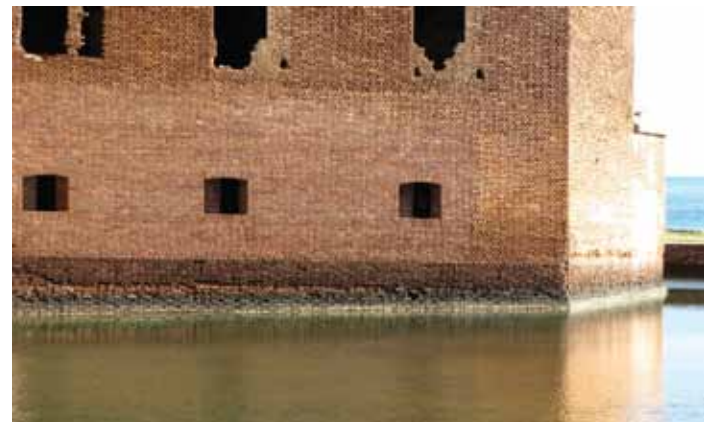
Figure 4: Settlements are as much as 24 inches per 200 feet. Here the water level in the moat makes settlement observation easy at Bastion 1.
