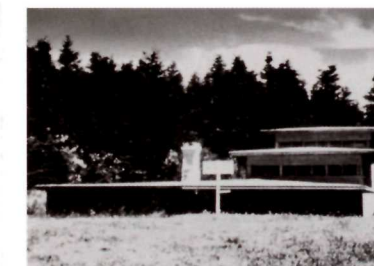
Fire Control Station
