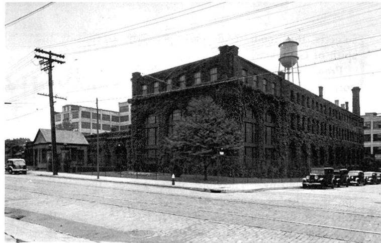
Main Laboratory and Gate House, 1939.
