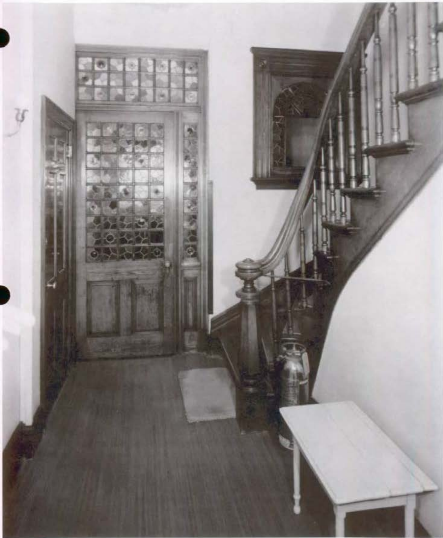
Figure 114. South part of Service Hall (Room 117), looking north, 1960.
