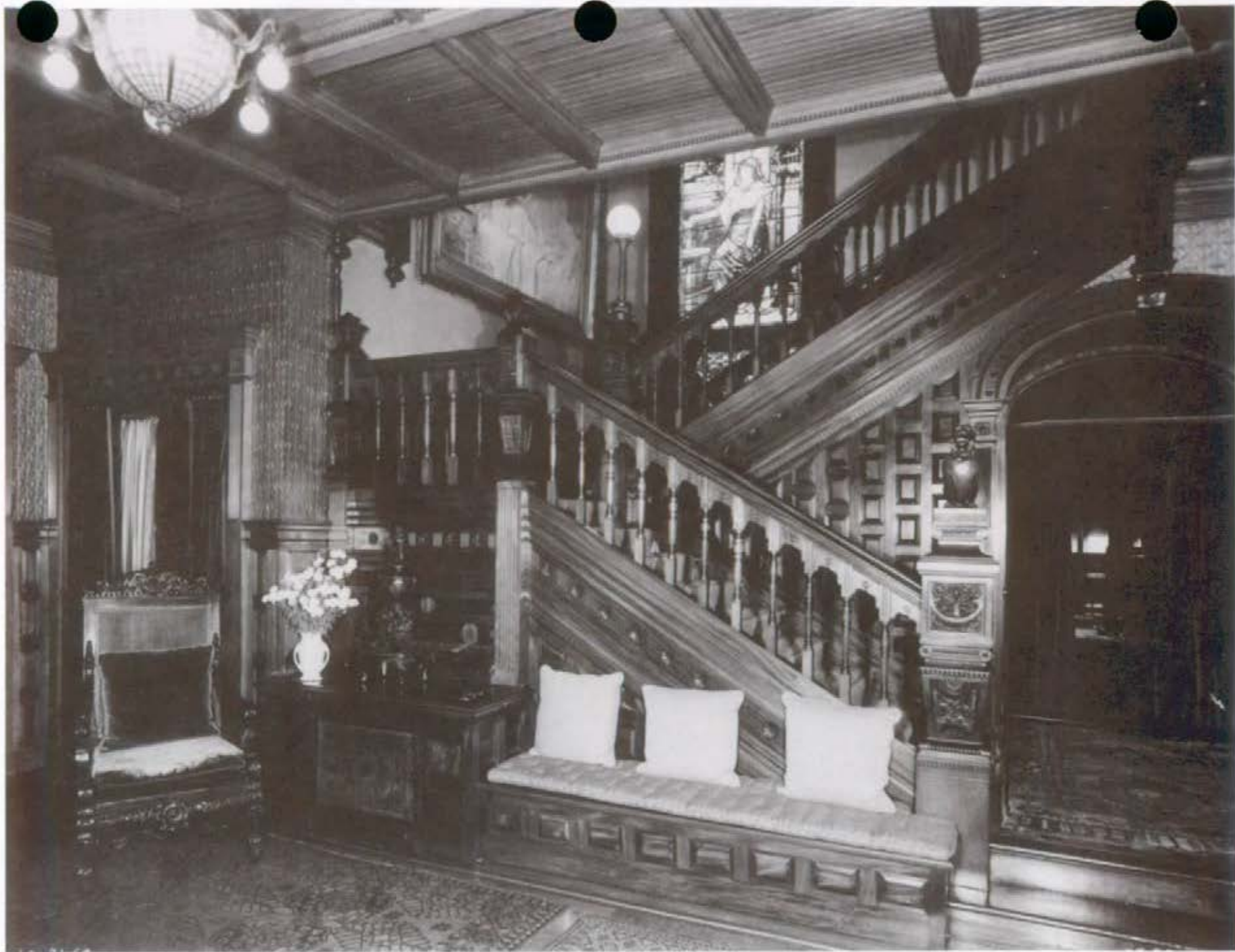
Figure 69. Hall (Room 103), looking west, 1960.
