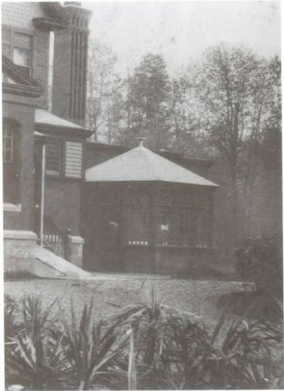
Figure 7. Detail of Figure 6, showing the "well house."
