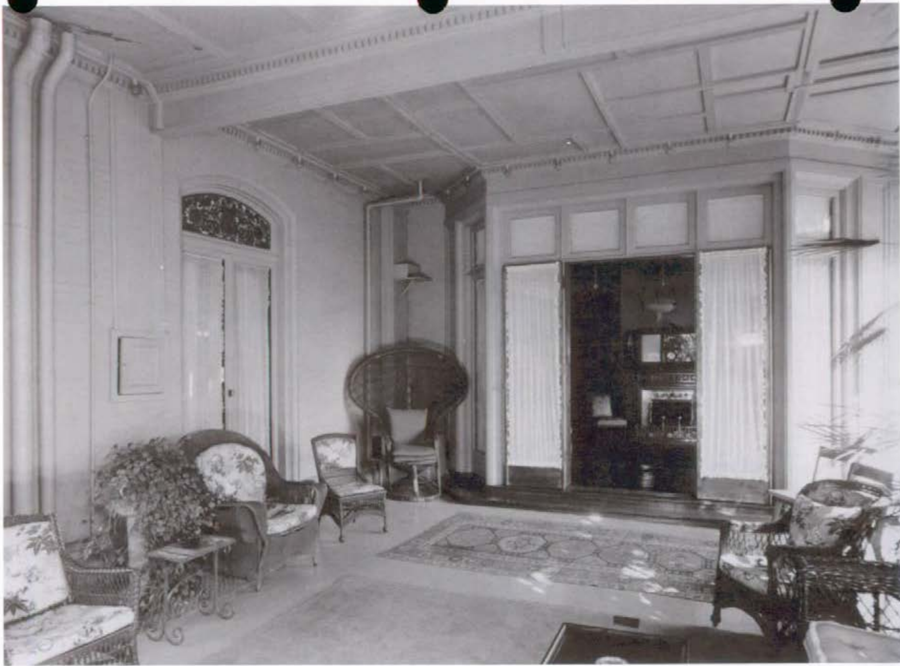
Figure 55. Conservatory (Room 101), looking northwest, 1960.
