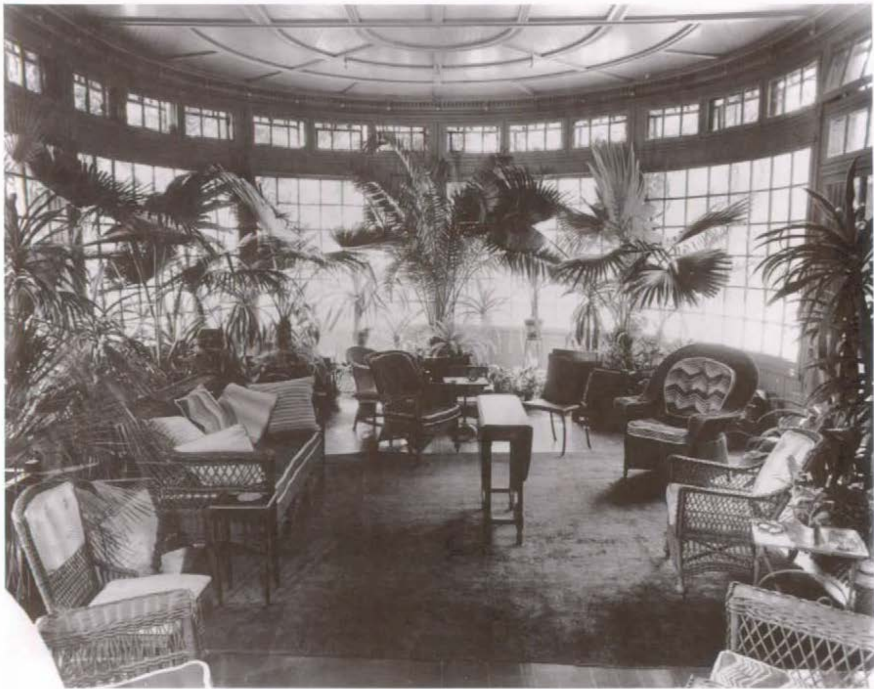
Figure 52. Conservatory (Room 101), looking south, 1947.
