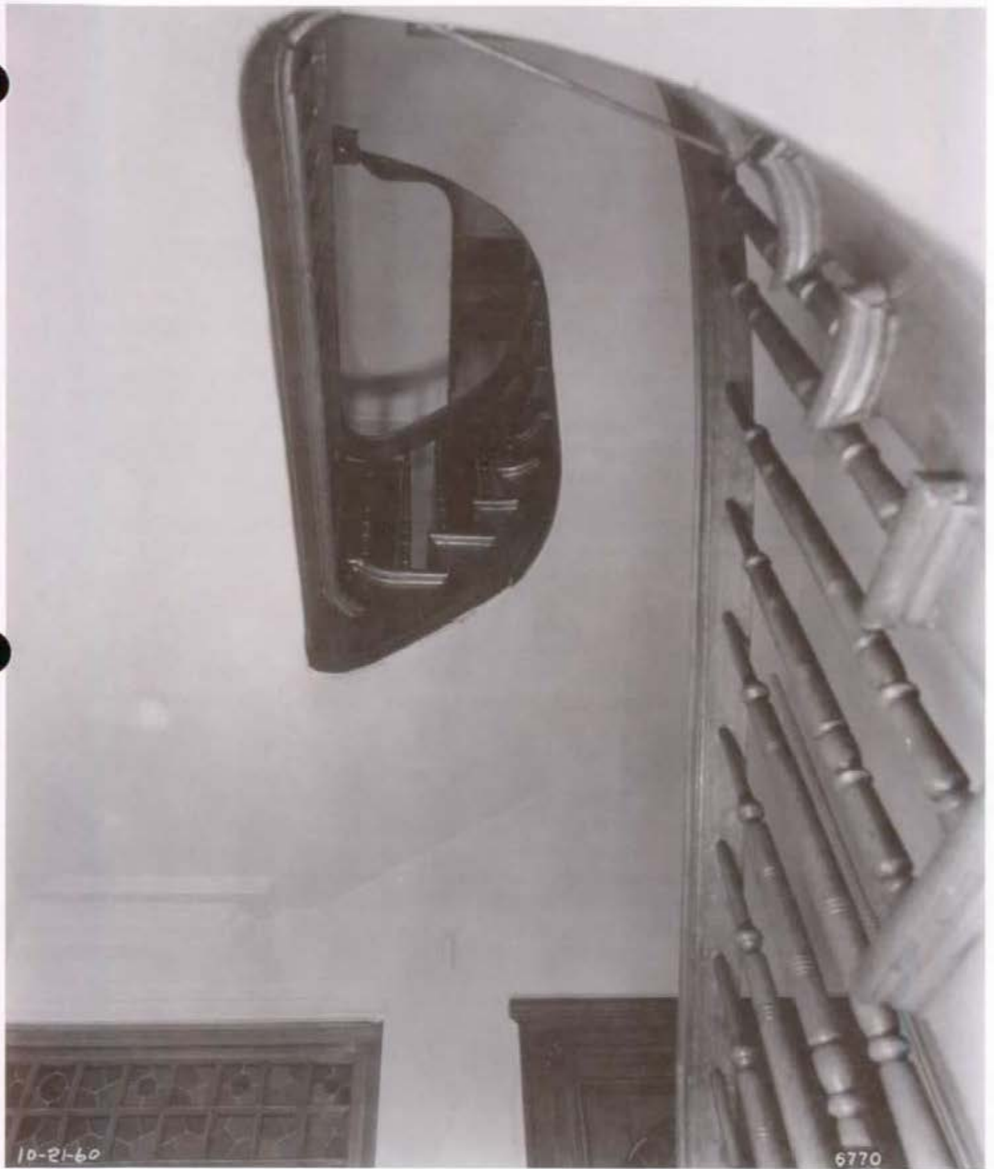
Figure 116. South part of Service Hall (Room 117), looking up at the Service Stairway, 1960.
