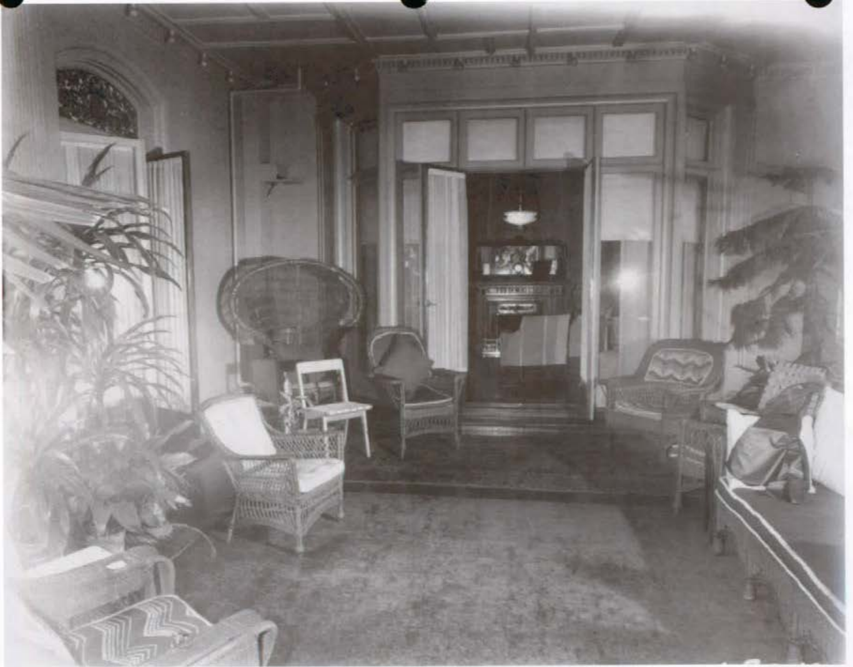
Figure 53. Conservatory (Room 101), looking northwest, 1947.
