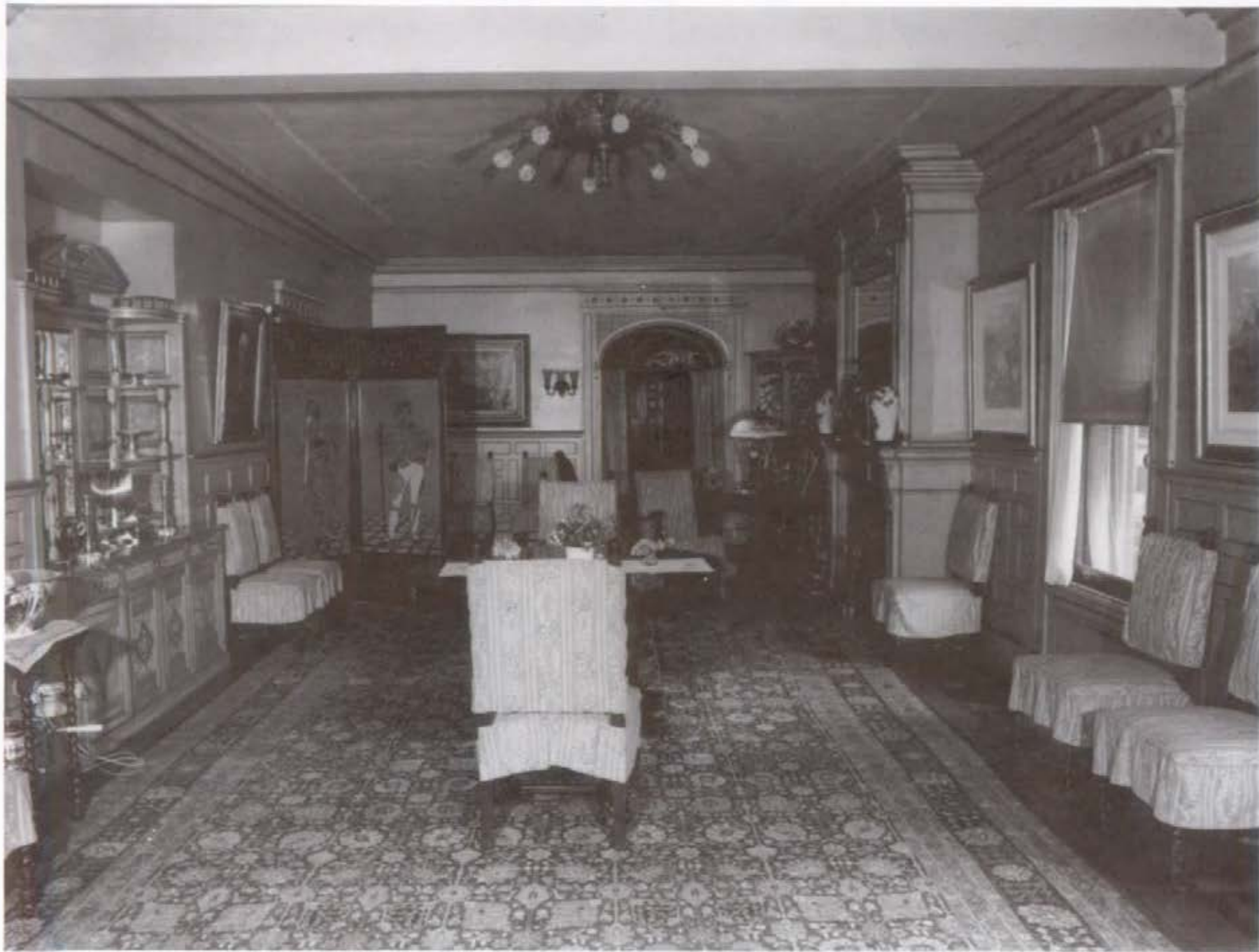
Figure 107. Dining Room (Room 115), looking east, 1947.
