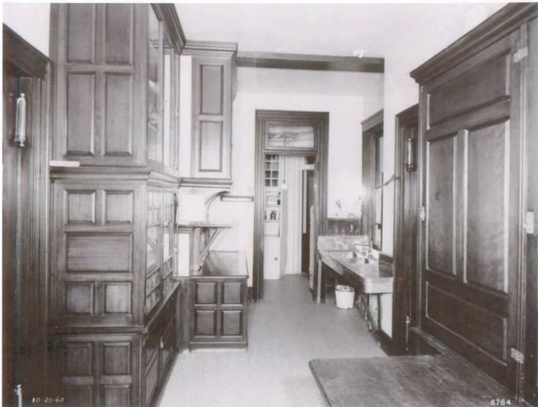
Figure 85. Pantry (Room 109), looking west, 1960.
