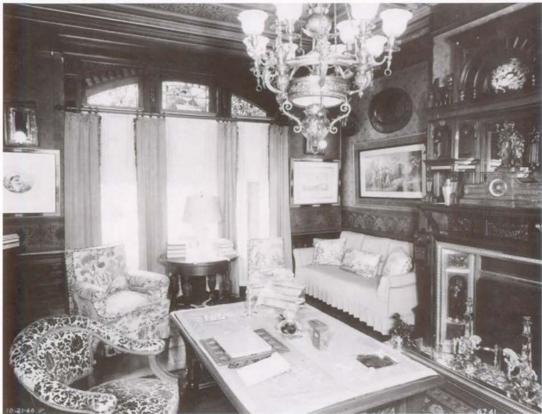
Figure 81. Library (Room 104), looking southeast, 1960.
