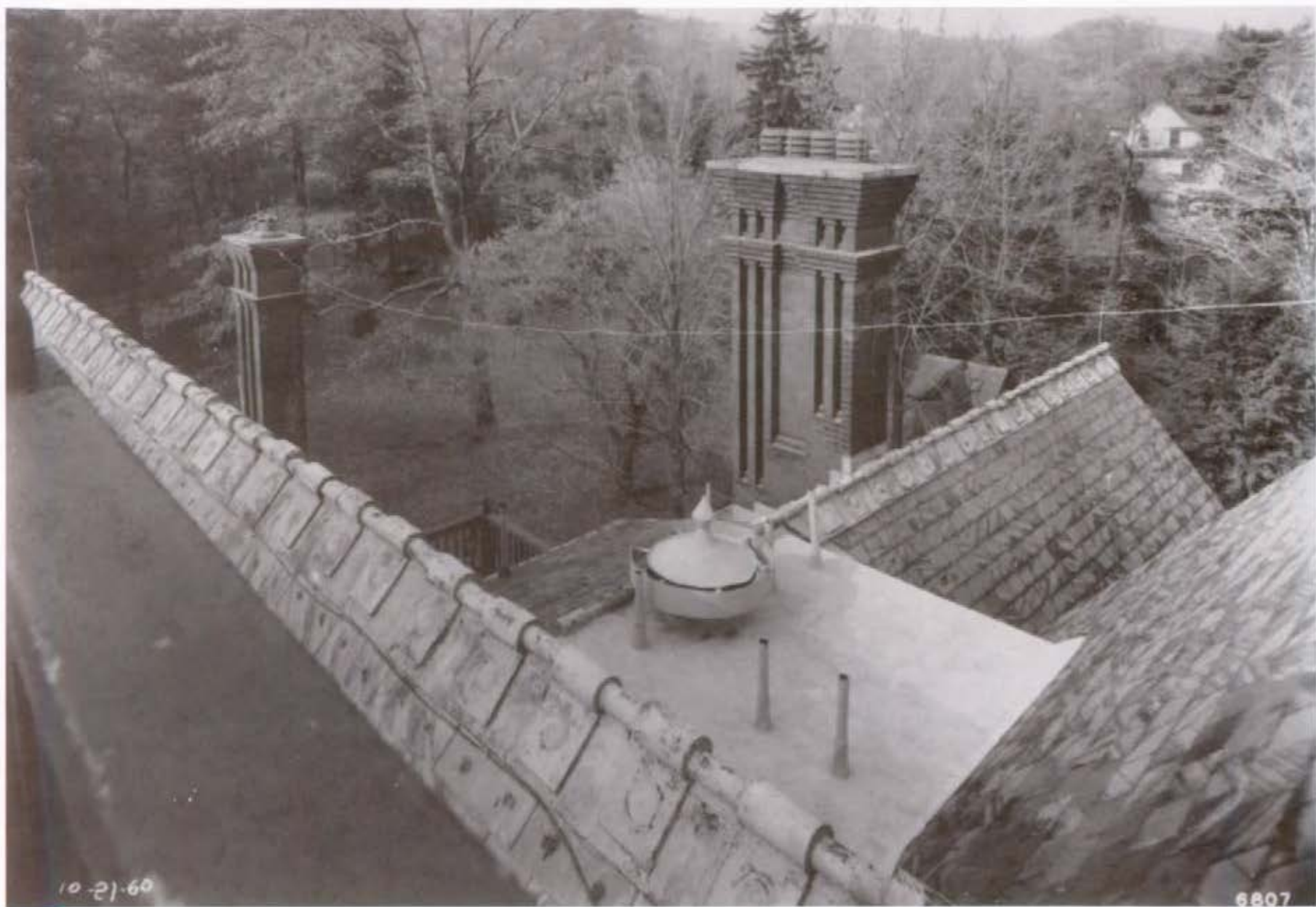
Figure 34. View of the roof, looking northwest, 1960.
