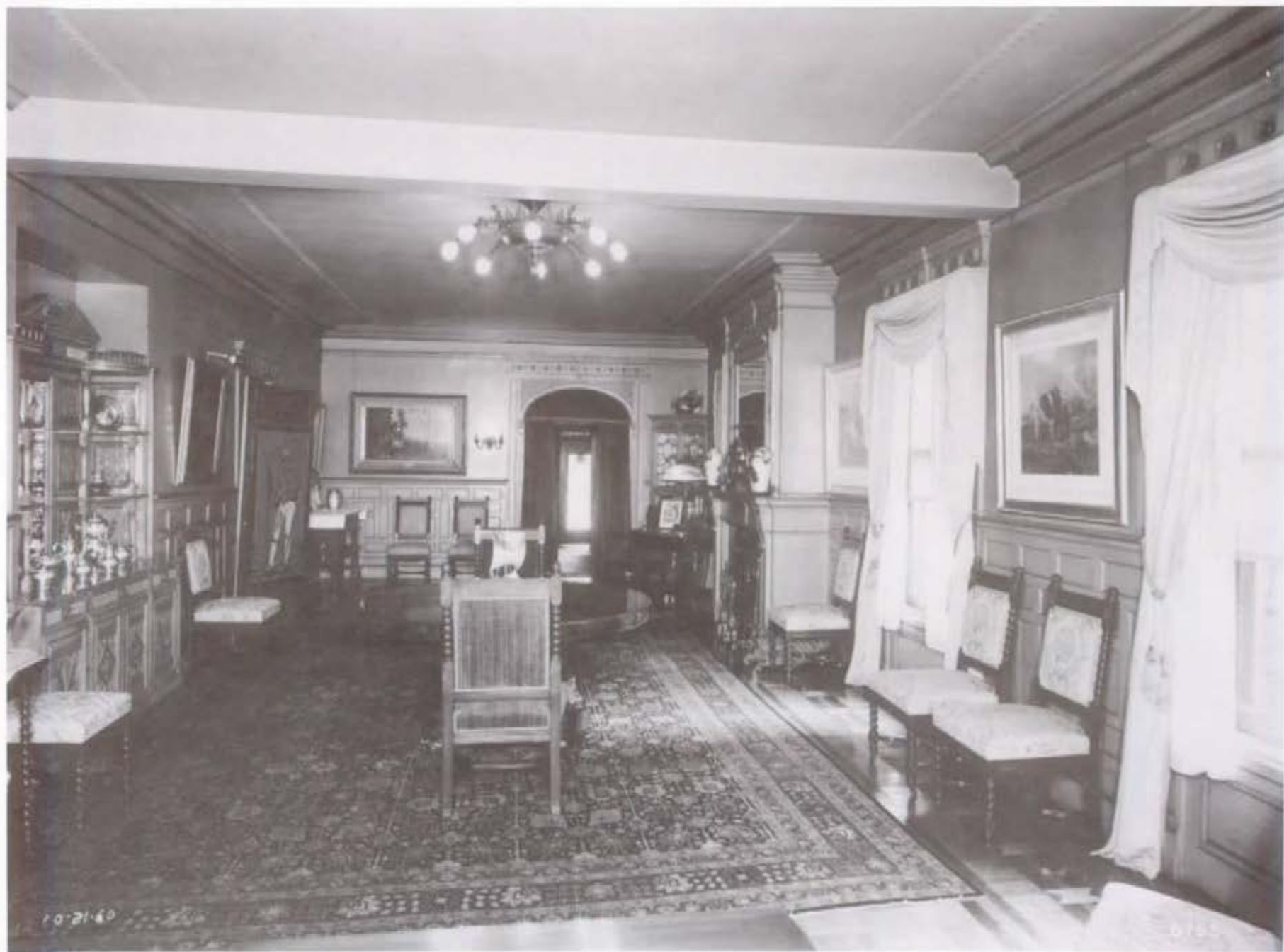
Figure 111. Dining Room (Room 115), looking east, 1960.
