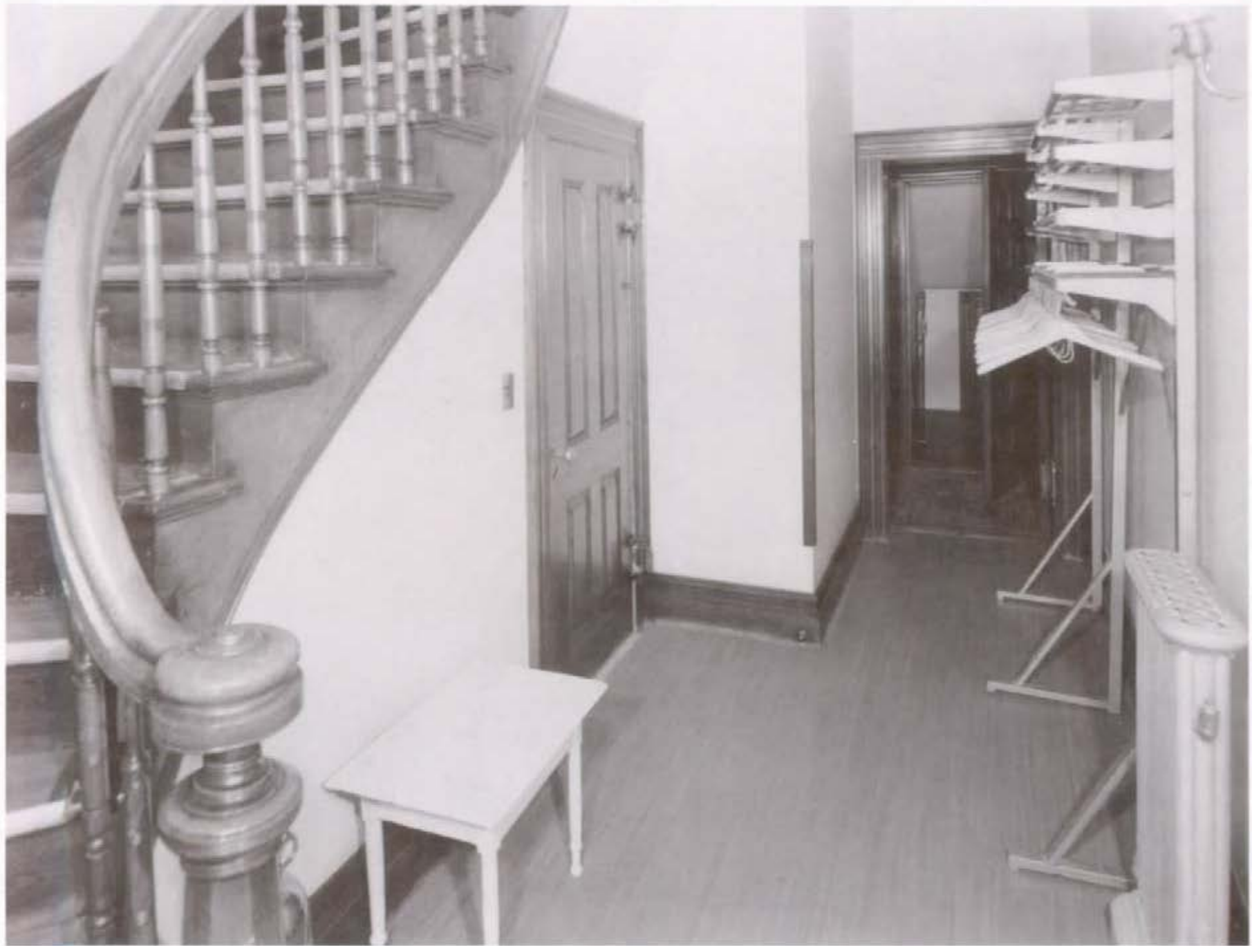
Figure 115. South part of Service Hall (Room 117), looking south, 1960.
