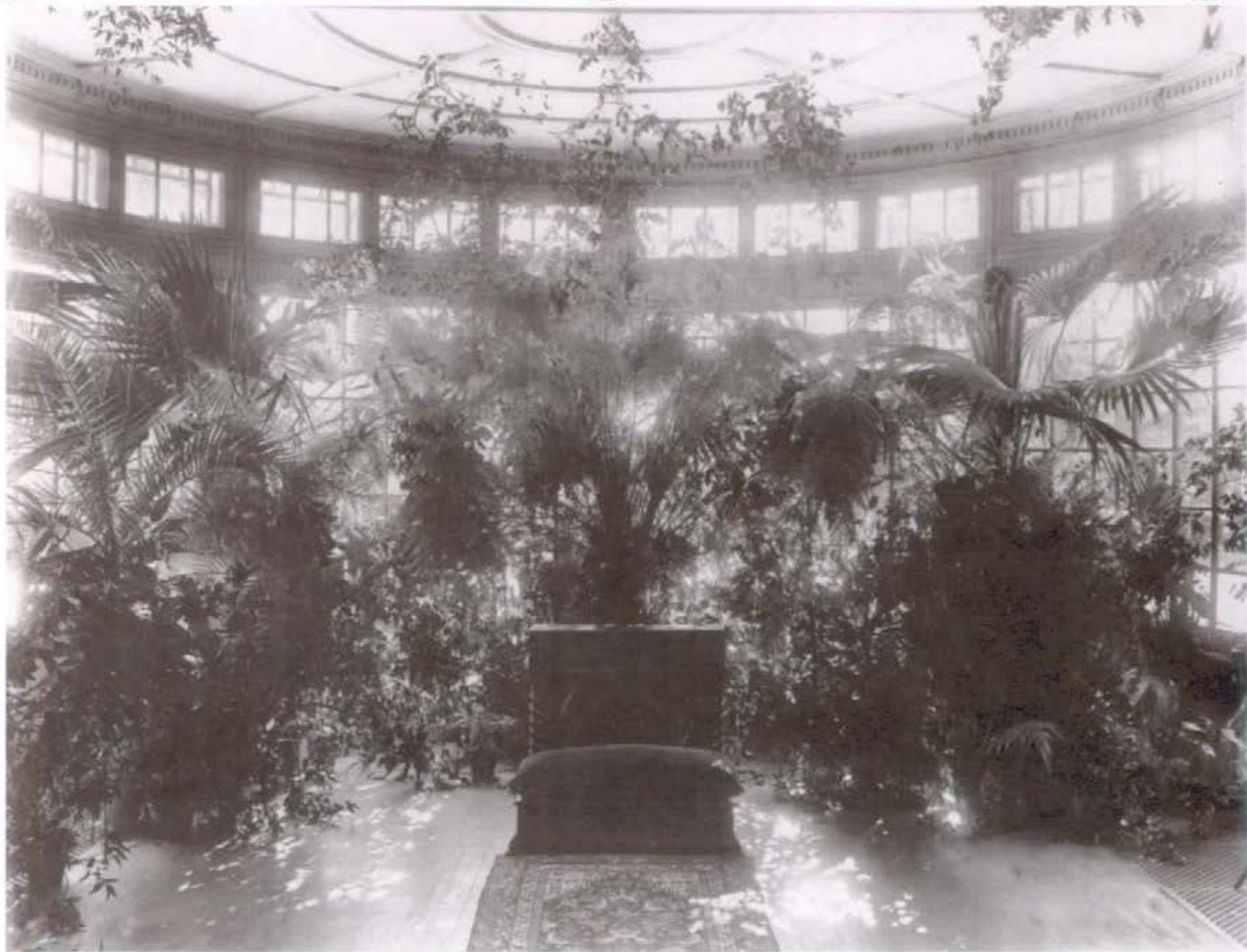
Figure 51. Conservatory (Room 101), looking south, 1916.
