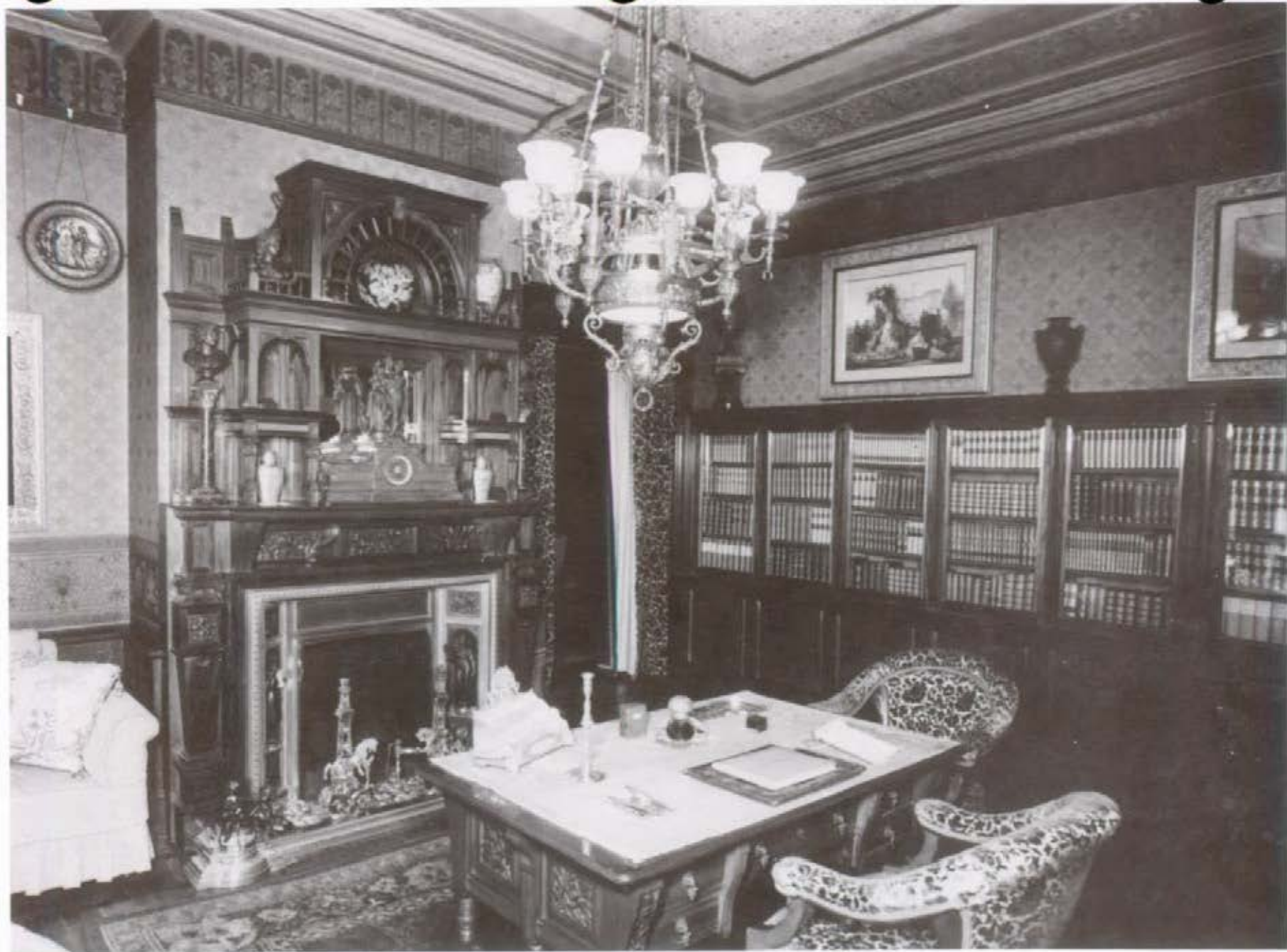
Figure 78. Library (Room 104), looking southwest, 1960.
