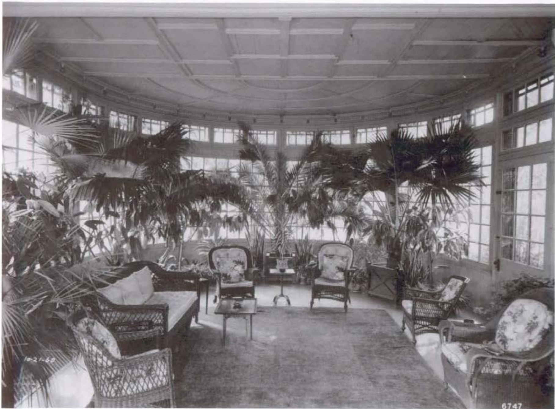
Figure 54. Conservatory (Room 101), looking south, 1960.
