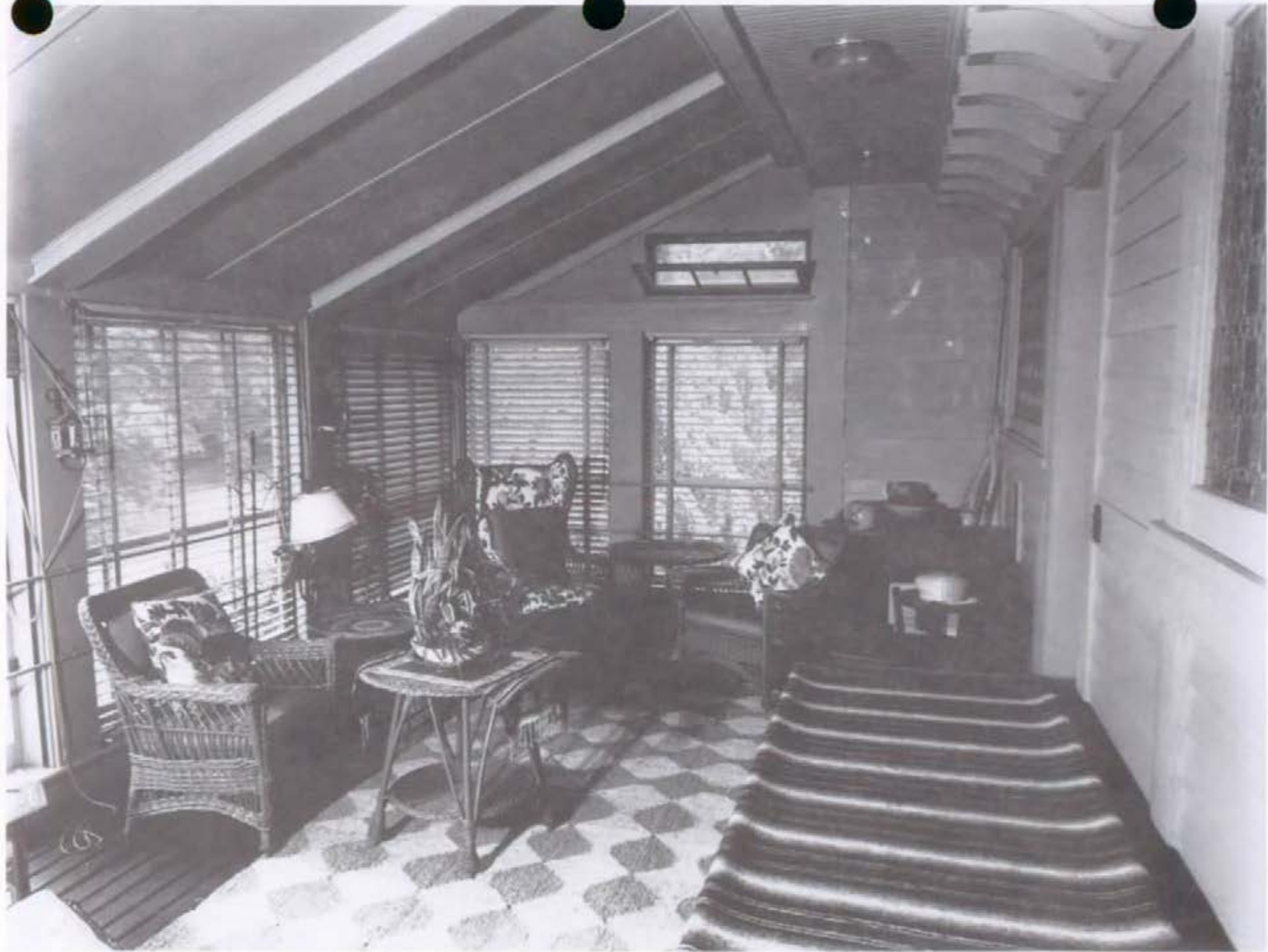
Figure 124. Second Story Porch (Room 202), looking west, 1947.
