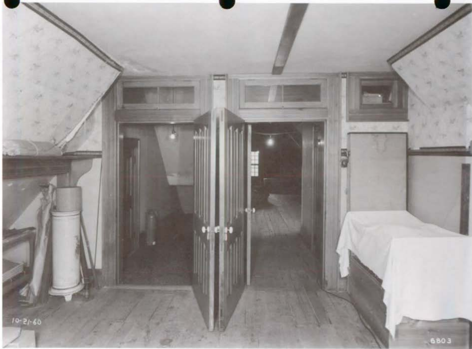
Figure 187. Bed Room (Room A1), looking north, 1960.
