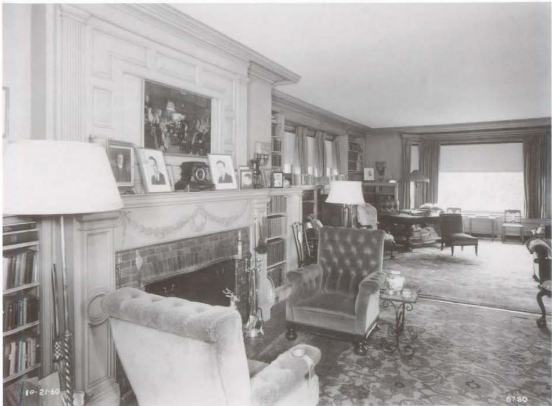
Figure 149. Living Room (Room 205), looking northeast, 1960.
