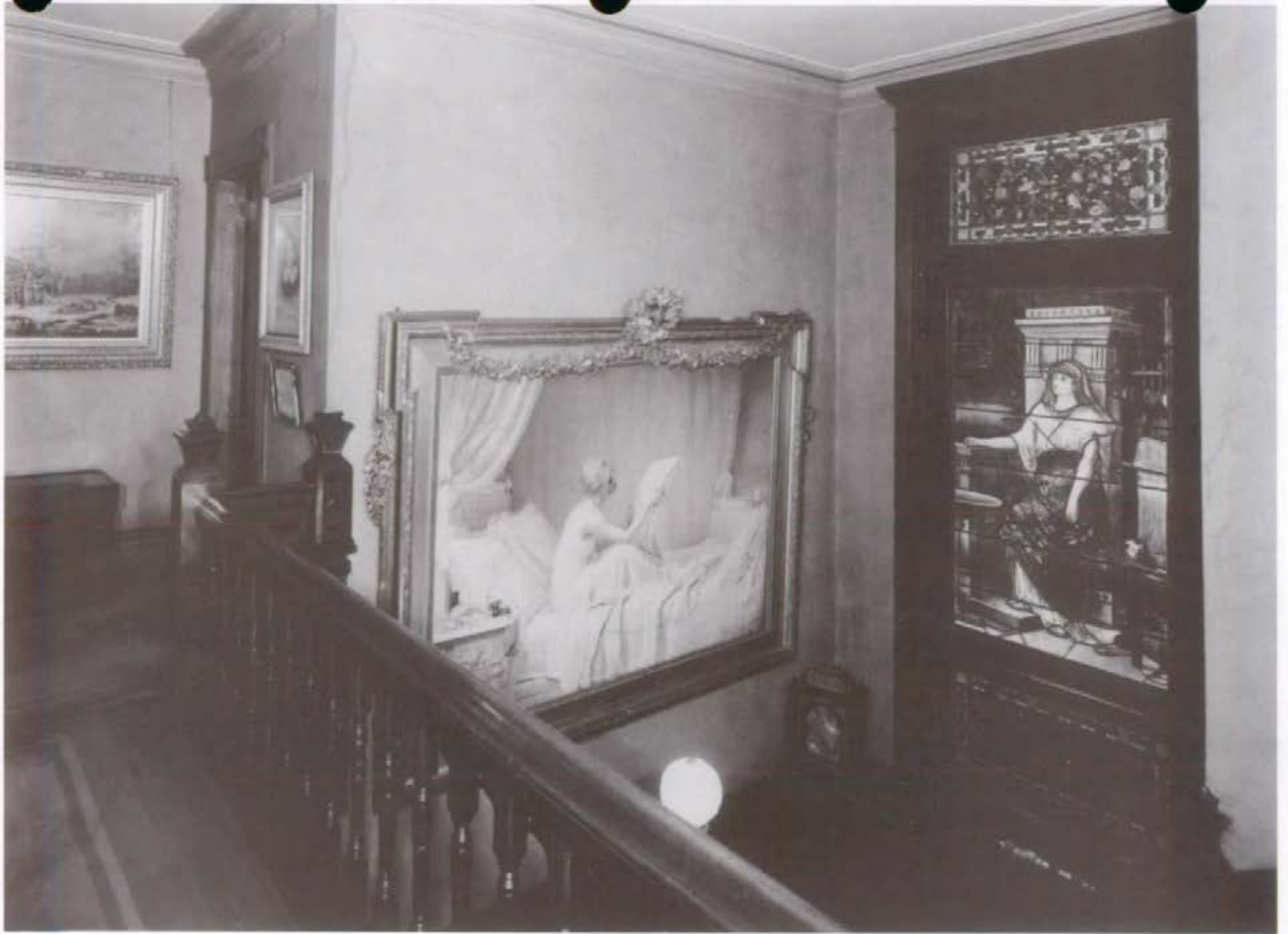
Figure 171. Second Floor Hall (Room 214), looking southwest, 1960.
