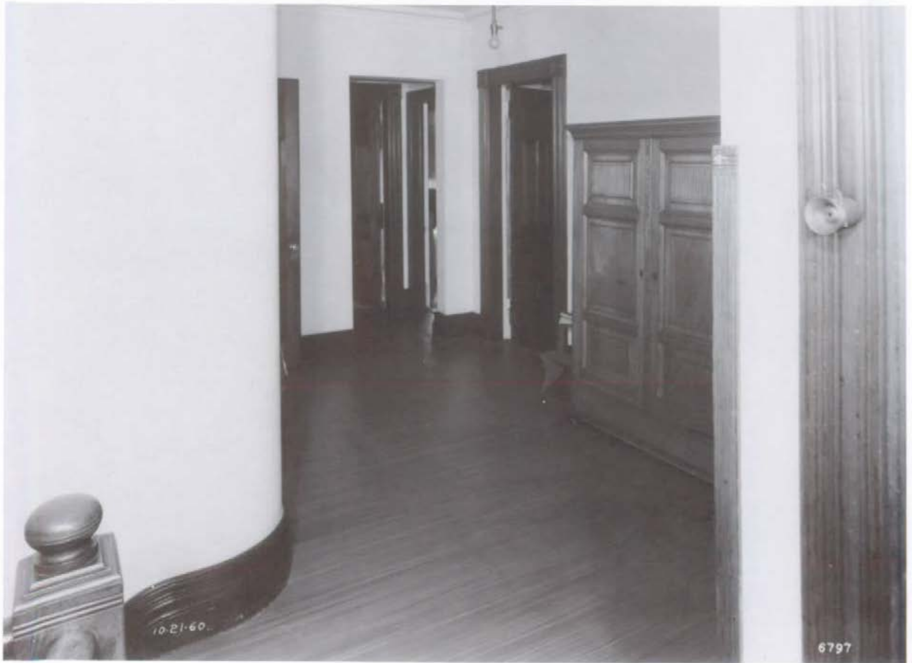
Figure 183. Hall: Service Port (Room 311), looking southwest, 1960.
