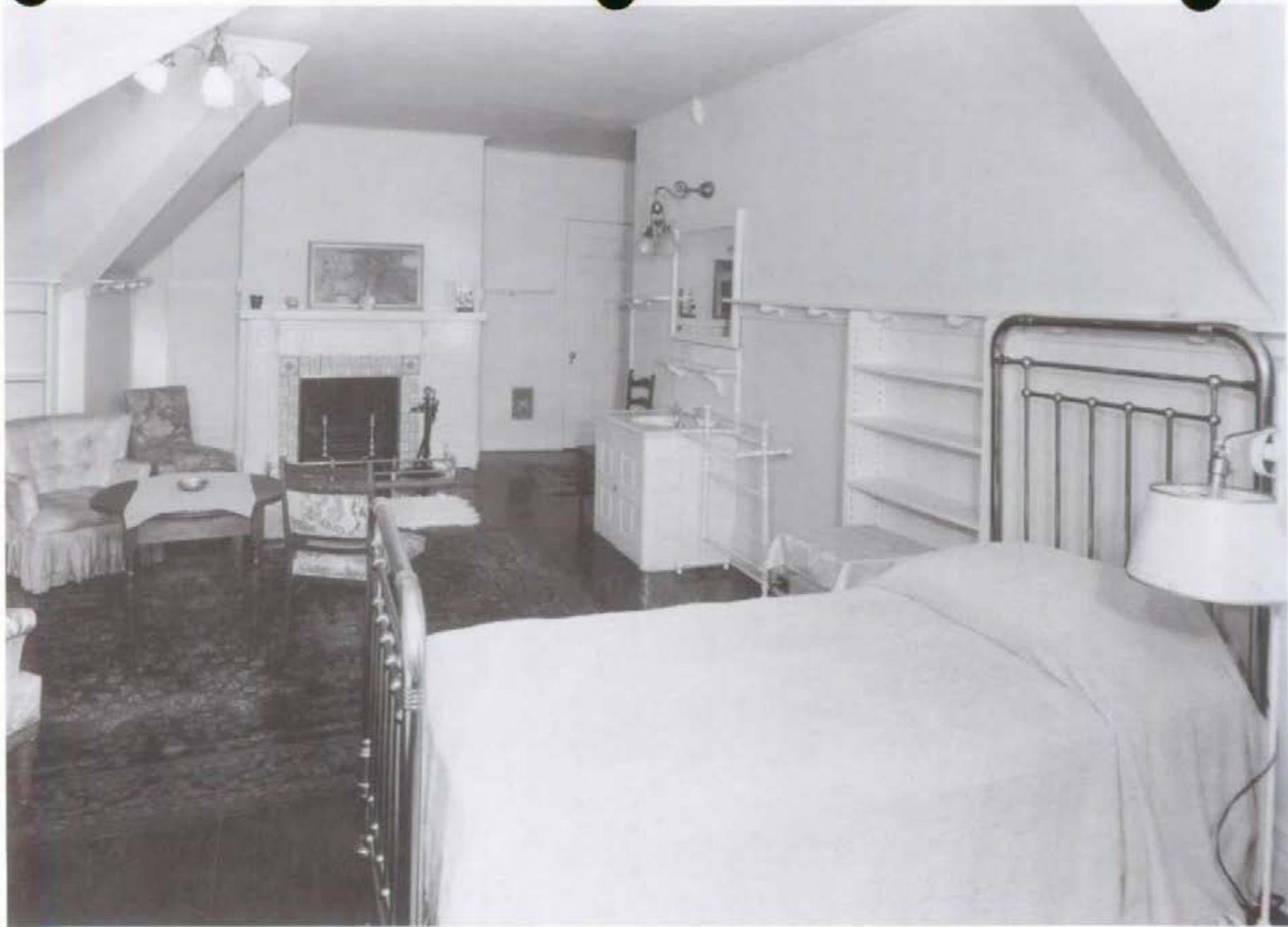
Figure 176. Mr. Charles' Room (Room 300), looking northeast, 1960.
