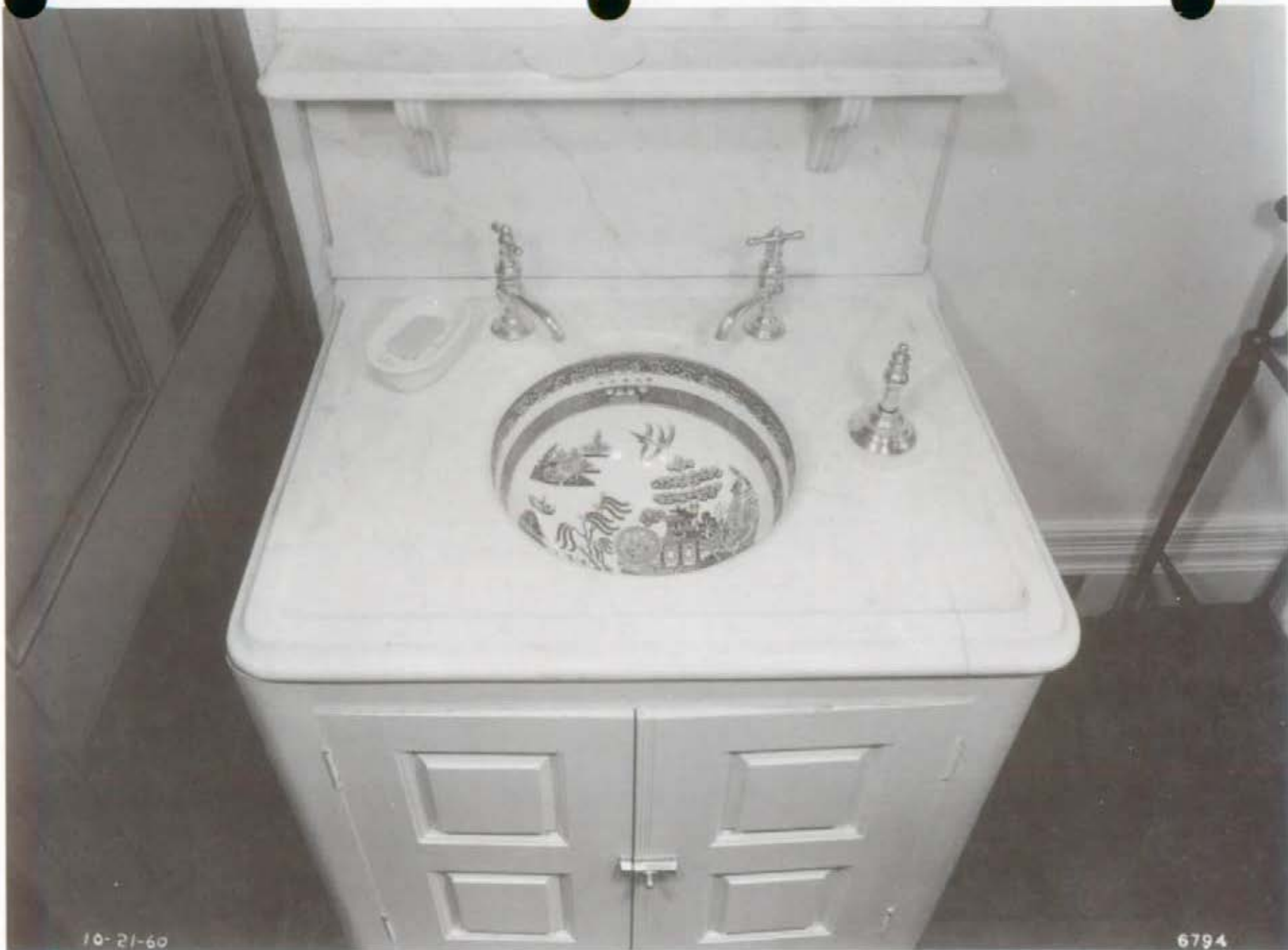
Figure 181. Sewing Room (Room 305), detail of marble-counter lavatory at the west wall, 1960.
