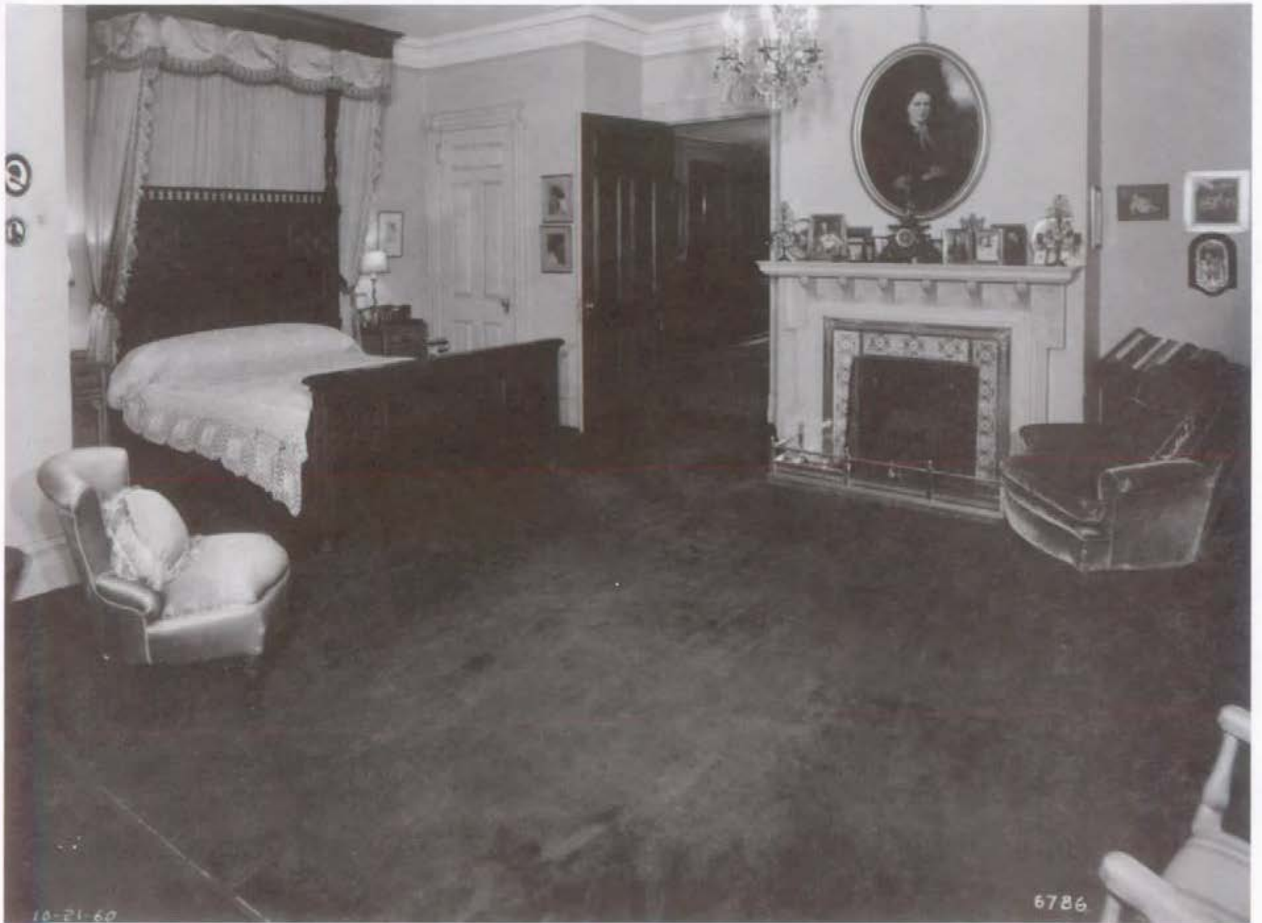
Figure 131. Owner's Room (room 203), looking northwest, 1960.
