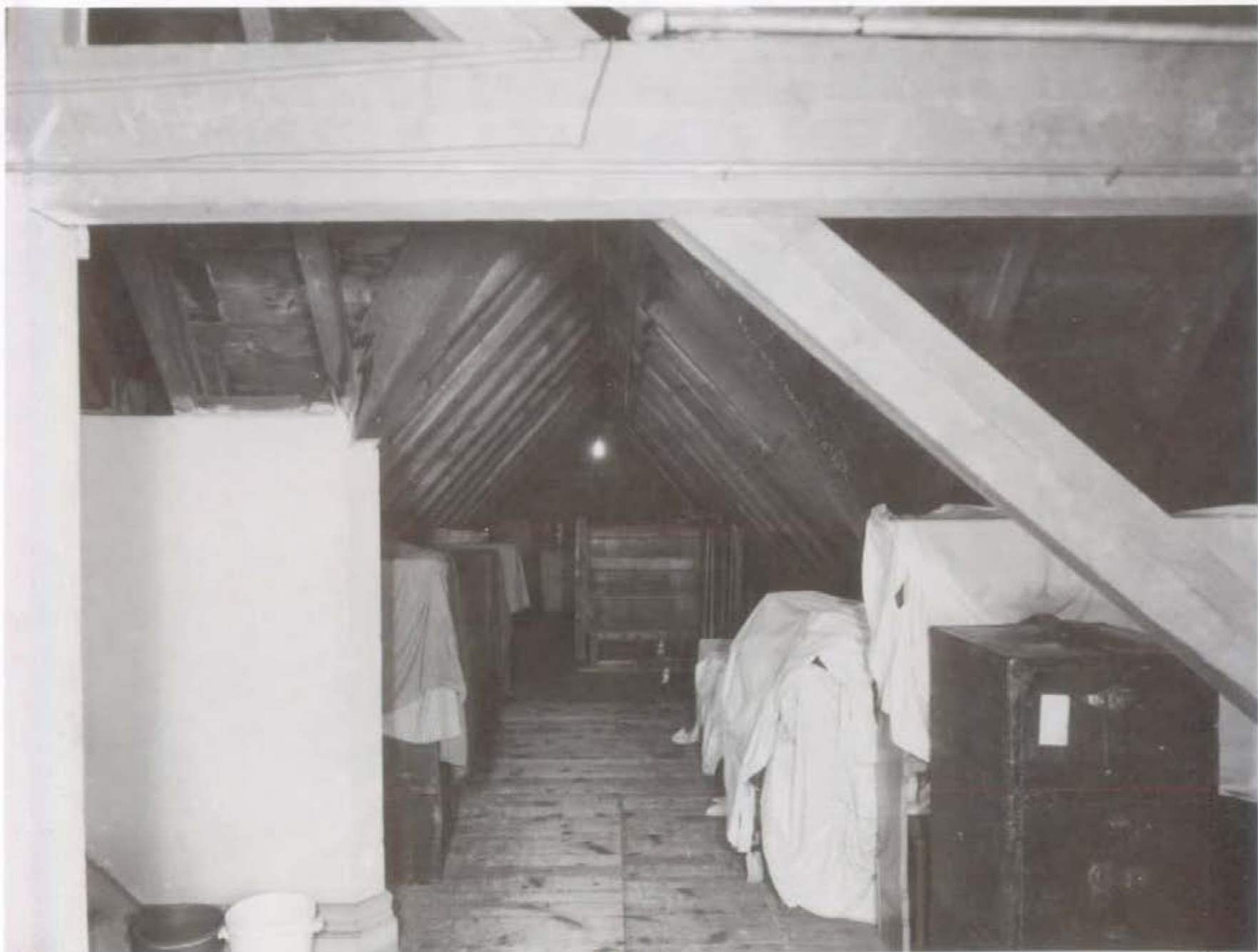
Figure 189. Unfinished Attic (Room A6), looking west, 1960.
