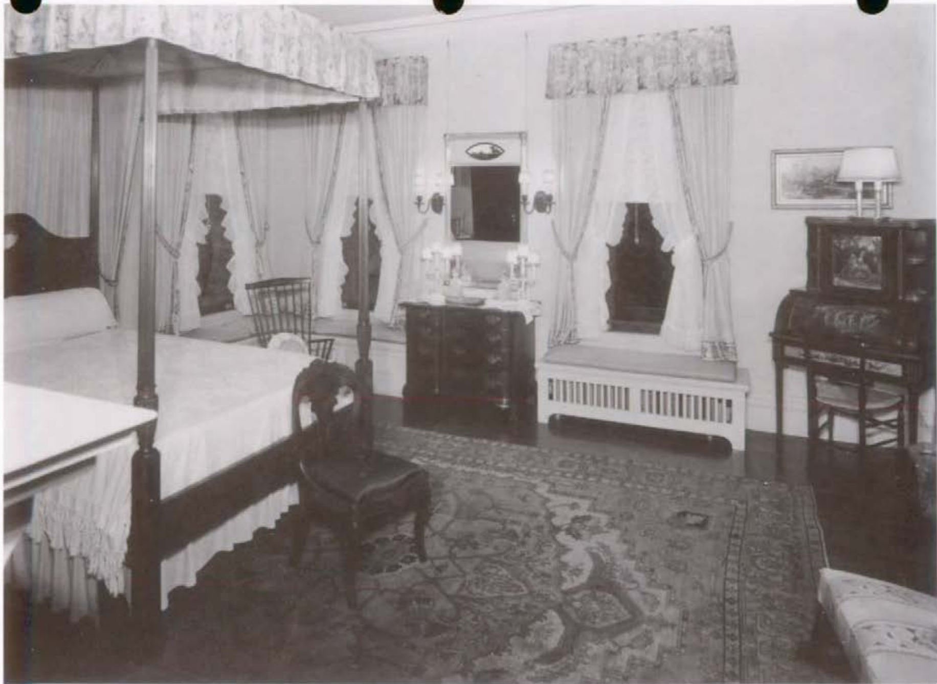
Figure 159. North Room (Room 210), looking northwest, 1960.
