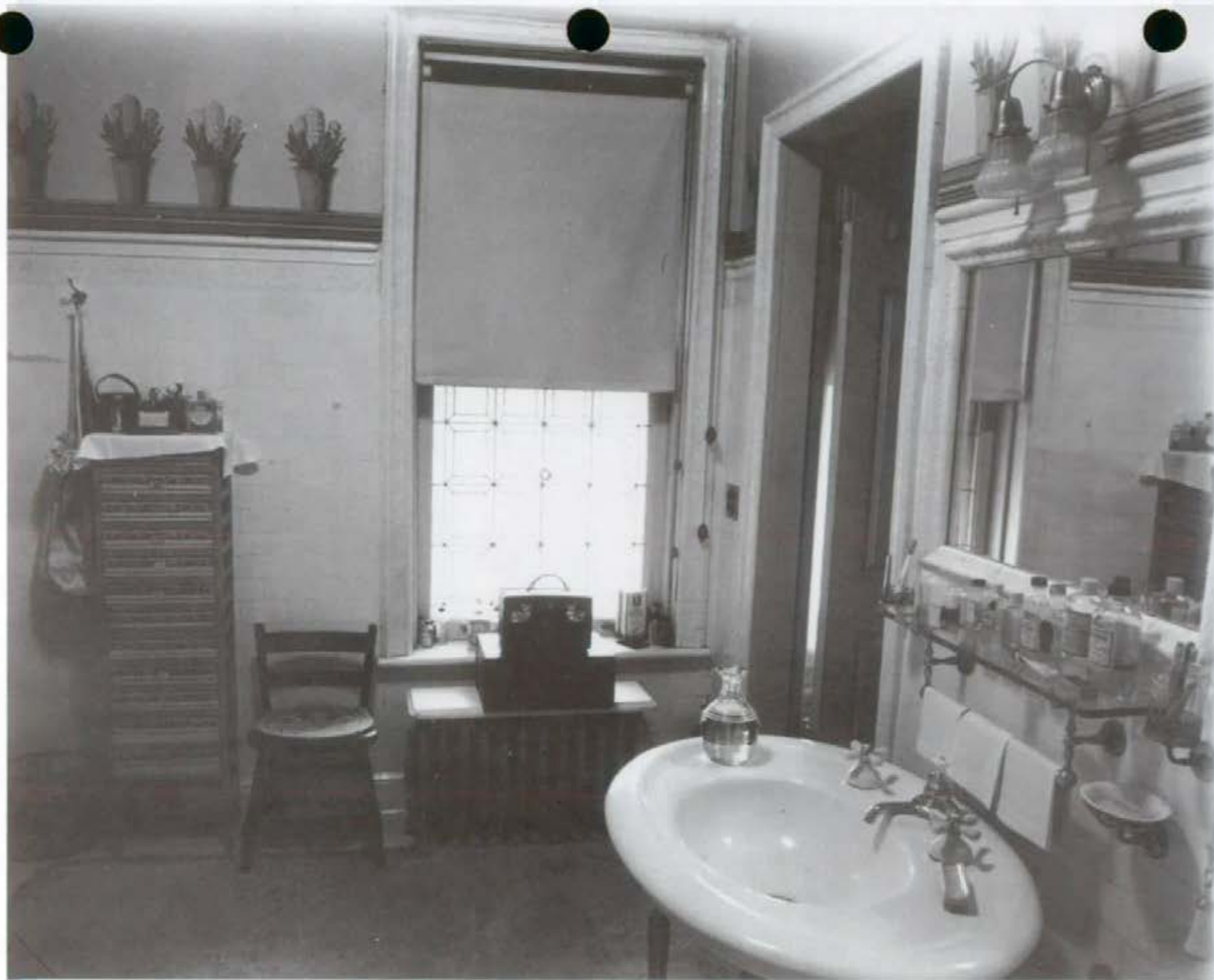
Figure 135. Owner's Bath (Room 204), looking southeast, 1947.
