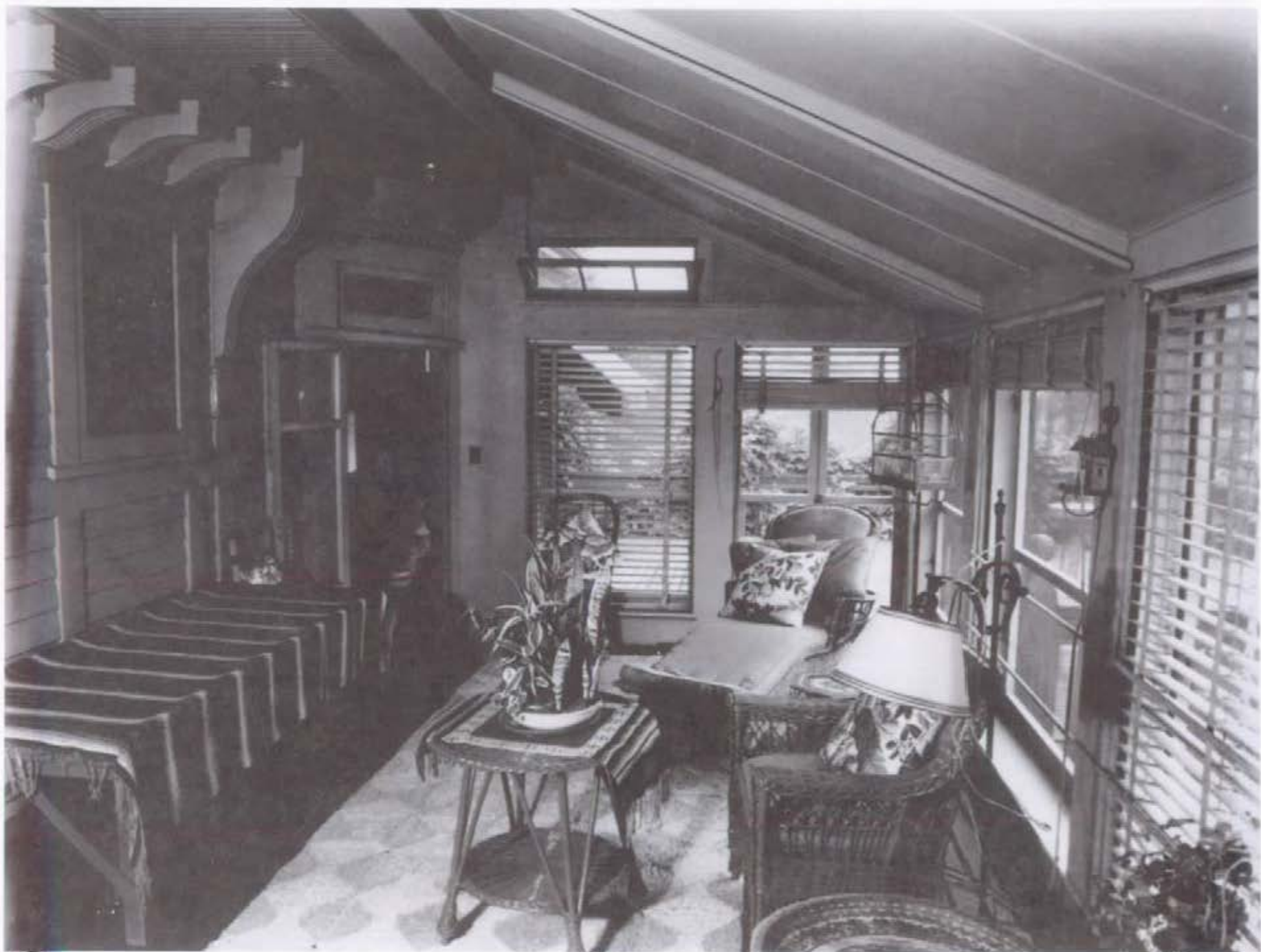
Figure 123. Second Story (Room 202), looking east, 1947.
