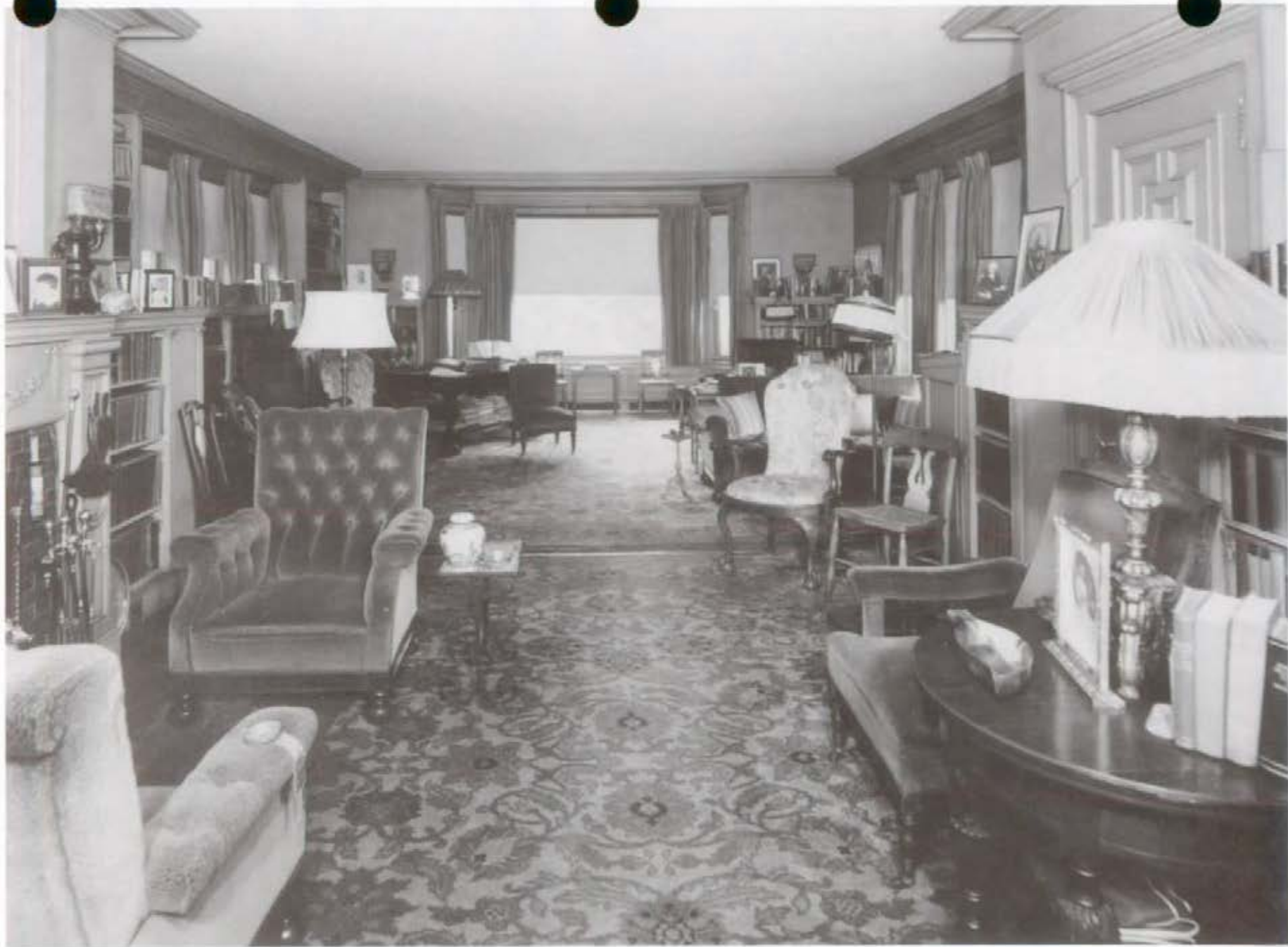
Figure 150. Living Room (Room 205), looking east, 1960.
