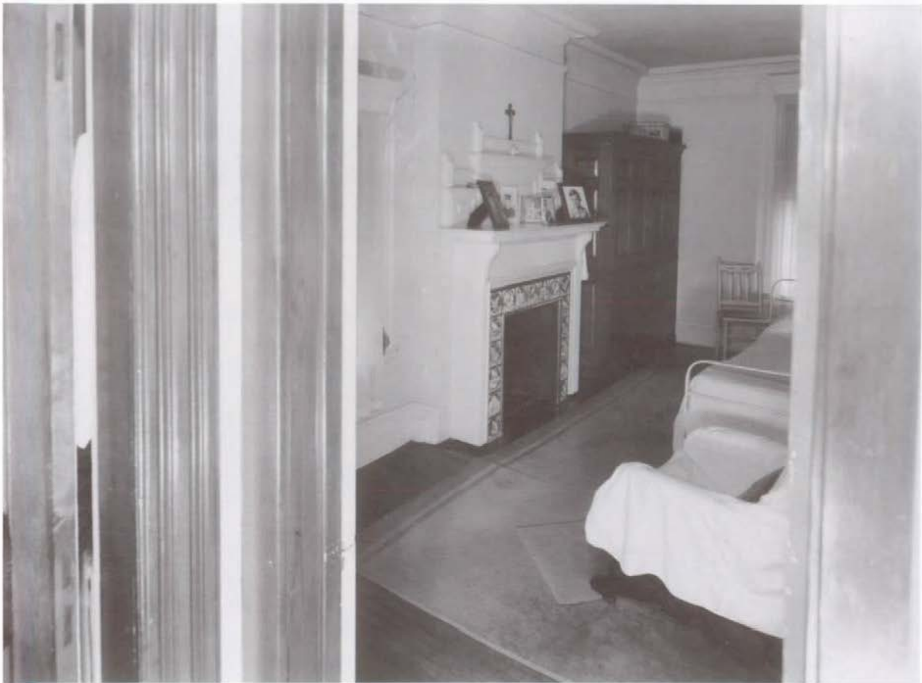
Figure 182. Bed Room #4 (Room 309), looking southwest, 1960.
