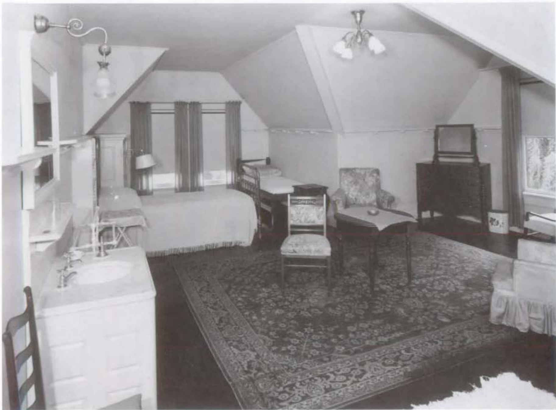
Figure 175. Mr. Charles' Room (Room 300), looking southwest, 1960.
