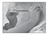
The inscriptions are carved into sandstone that is very weakly cemented—the sand particles are held together only by clay between the grains. The poor cementation of the rock made it easy to carve inscriptions, but it is also the reason the rock is deteriorating quickly.
