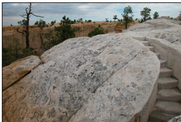
Figure 29. Steps carved into Zuni Sandstone. To facilitate access to the mesa top, the Civil Works Administration carved steps into the top of the Zuni Sandstone in the 1930s. These steps cut into the bleached horizon. The steps impact natural runoff during storms, but are a significant cultural resource and preserved by the National Park Service. Note the jointed walls of the box canyon in the background. National Park Service photograph by Sarah Beckwith.
