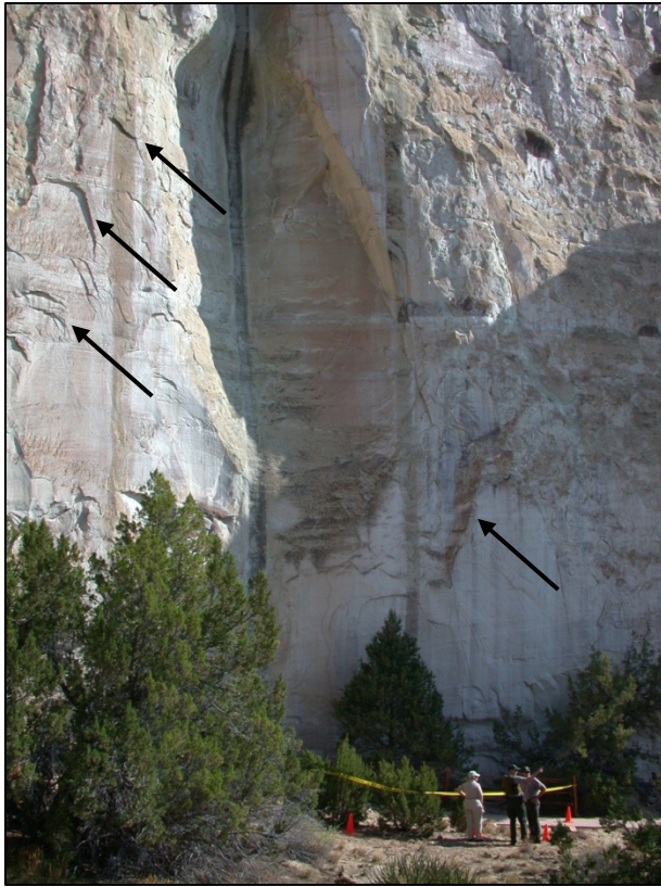
Figure 10. Cliffs above Inscription Rock Trail. Areas prone to rockfall include the cliffs above Inscription Rock Trail. The trail is visible in the photograph at the base of the cliff, behind park staff. At the time the photograph was taken, the trail was closed as a result of a rockfall event on 27 June 2006. Management concerns include visitor safety, loss of inscriptions, and damage to the existing trail. Arcuate “lips” of rock with smooth rock faces below indicate areas where slabbing has occurred (arrows; see also fig. 12). National Park Service photograph.
