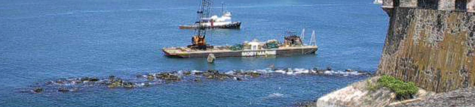
A barge conducts an emergency repair on a protective breakwater at El Morro Castle, San Juan National Historic Site that was damaged by the grounding of a large ship.
