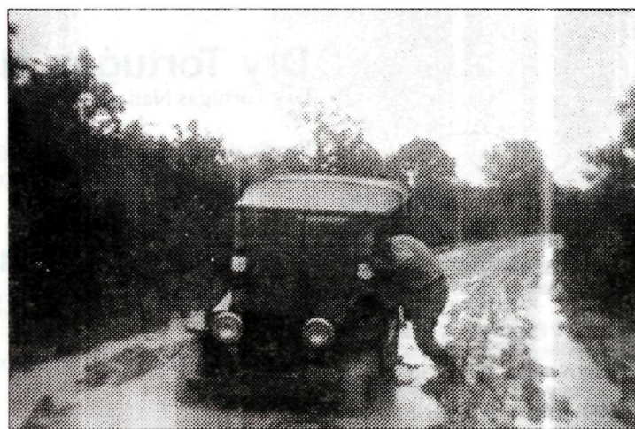
Early roads into the Everglades were hardly roads at all. Still, they were quite effective at altering the natural flow of water.
