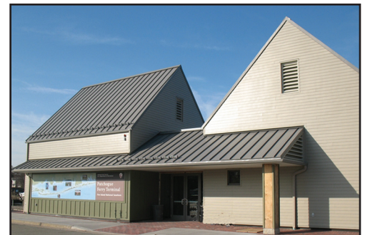
The new Patchogue Ferry Terminal.
