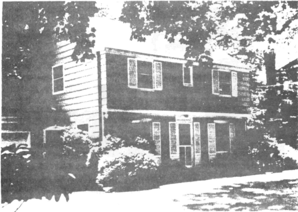
Garrison House Colonial Second story protrudes in front, House is otherwise symmetrical
