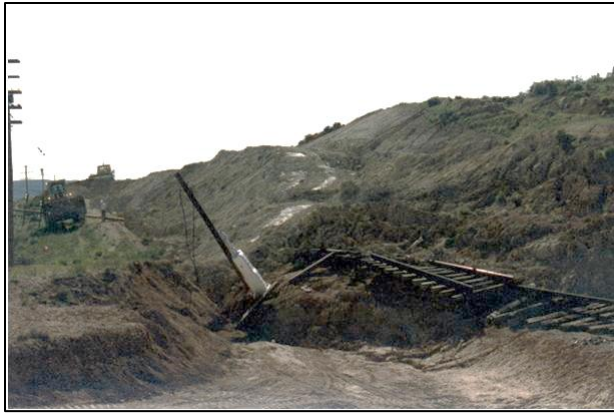
Figure 12. Landslide damage. In 1984, a massive landslide on the southeastern flank of Fossil Butte destroyed a portion of the Union Pacific Railroad line immediately adjacent to the park boundary. Left view is to the west, right view is to the east. National Park Service photographs.
