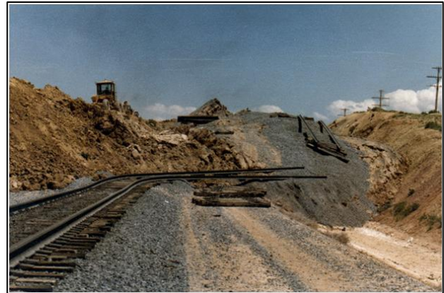
Figure 12. Landslide damage. In 1984, a massive landslide on the southeastern flank of Fossil Butte destroyed a portion of the Union Pacific Railroad line immediately adjacent to the park boundary. Left view is to the west, right view is to the east. National Park Service photographs.
