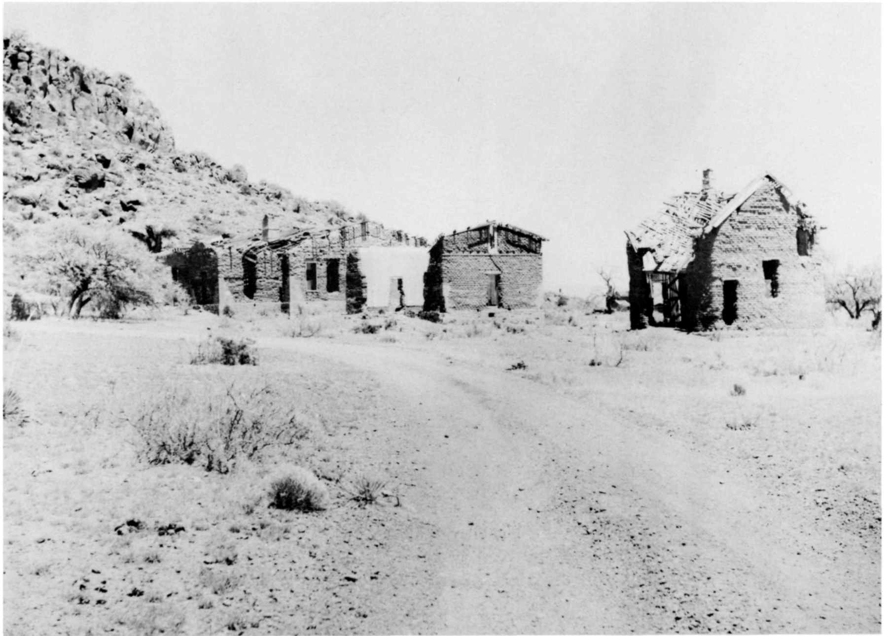
Hospital and quarters of Hospital Steward, looking northeast. NPS photo, April 1960.
