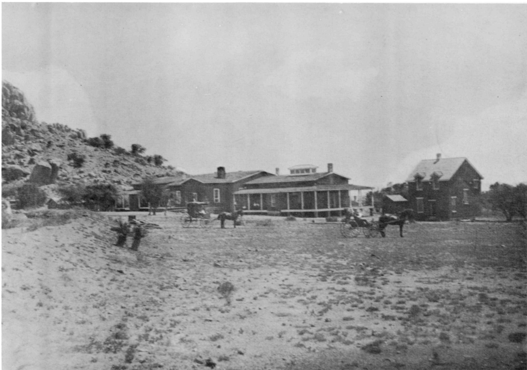
Hospital and Hospital Steward's Quarters, Fort Davis, about 1885. From glass plate owned by Mrs. John C. Jackson, Houston, Texas.
