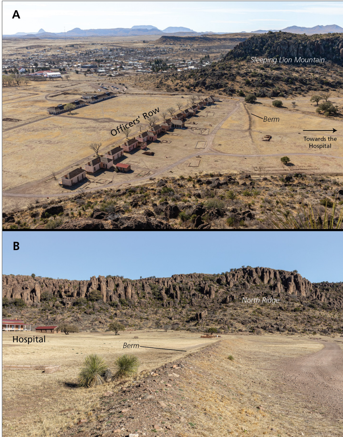
Figure 11. Photographs of the berm between the hospital and Officers' Row. The berm was built to limit water flow into the main section of the fort. A) Officers' Row, the line of houses, spans across the entrance to Hospital Canyon. The berm exists west of Officers' Row. Water can get trapped behind the berm, resulting in flooding toward the hospital. Sleeping Lion Mountain can be seen towering over the fort in the background. B) A close-up view of the berm as of 2023. The hospital can be seen in the background at the side of the photo. Photos by Matthew Harrington (Colorado State University).
