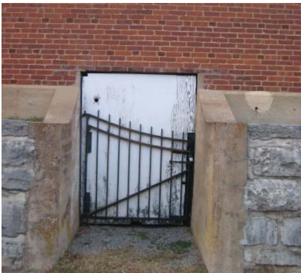
Figure 68. Iron gate at entrance to Basement.
