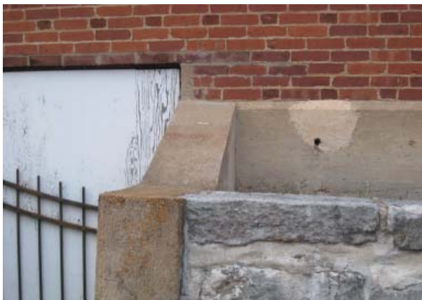
Figure 77. Exterior patch over flue opening in south wall.
