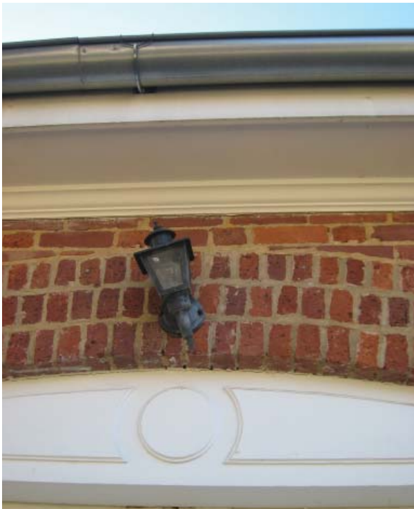
Figure 51. Typical carriage light exterior fixture.
