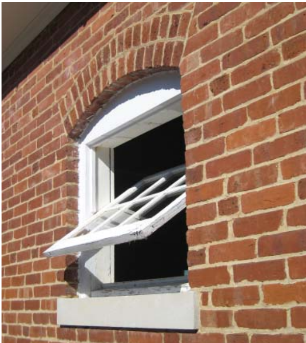
Figure 61. Pivot window, exterior view.
