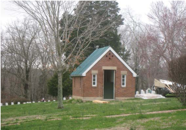
Figure 111. East elevation during construction. (FODO collection)
