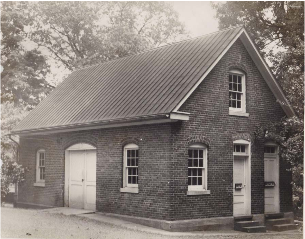
Figure 19. Undated photograph shows entrances to men's and women's restrooms at west gable end. Modification in brickwork indicates conversion of center window to doorway. (FODO collection)
