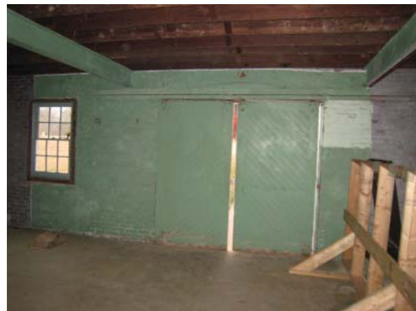
Figure 88. North wall of center section.
