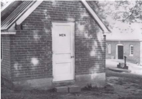
Figure 107. West gable end shown in 1964. Note the change in grade, awkward step, and absence of paved walkway. Roof hatch above the well is visible on north slope. Carriage House/Stable is in background. (FODO collection)
