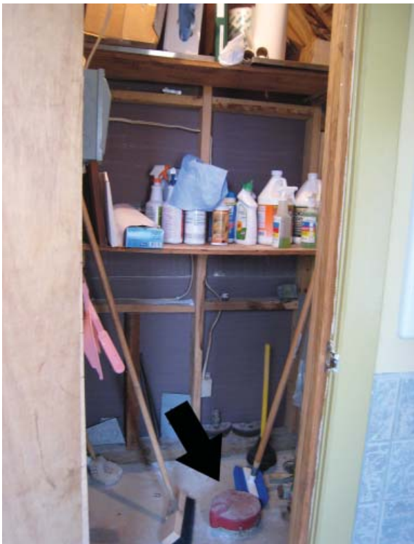
Figure 137. West wall of Service Closet and wellhead at floor.
