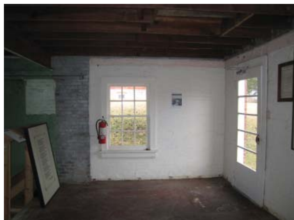
Figure 80. North wall of east section.
