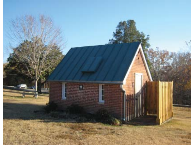
Figure 112. North elevation of the Pump House in 2010.
