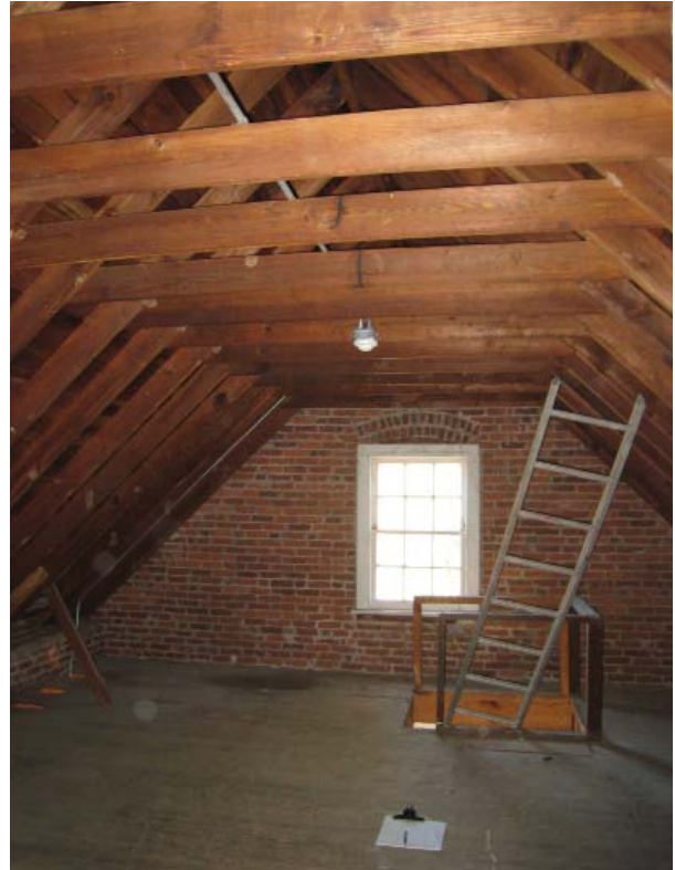
Figure 103. West gable wall.
