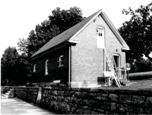
Figure 30. 1974 photograph showing east and south elevations, replacement steps at east entrance. (National Register nomination)
