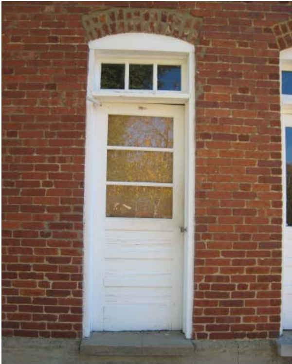
Figure 67. Added central doorway of west elevation.
