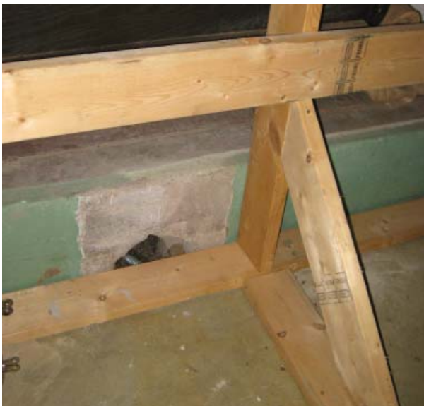
Figure 87. An 8" diameter hole at raised floor.
