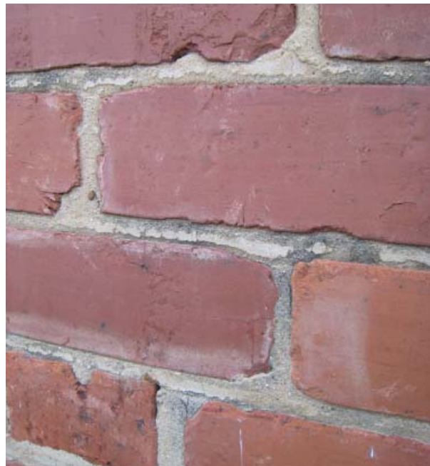
Figure 35. Decorative penciling of mortar joints.
