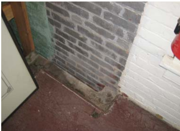
Figure 84. Slot cast in northwest corner of raised floor.
