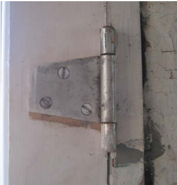
Figure 97. Modern barn-type strap hinge on south door.
