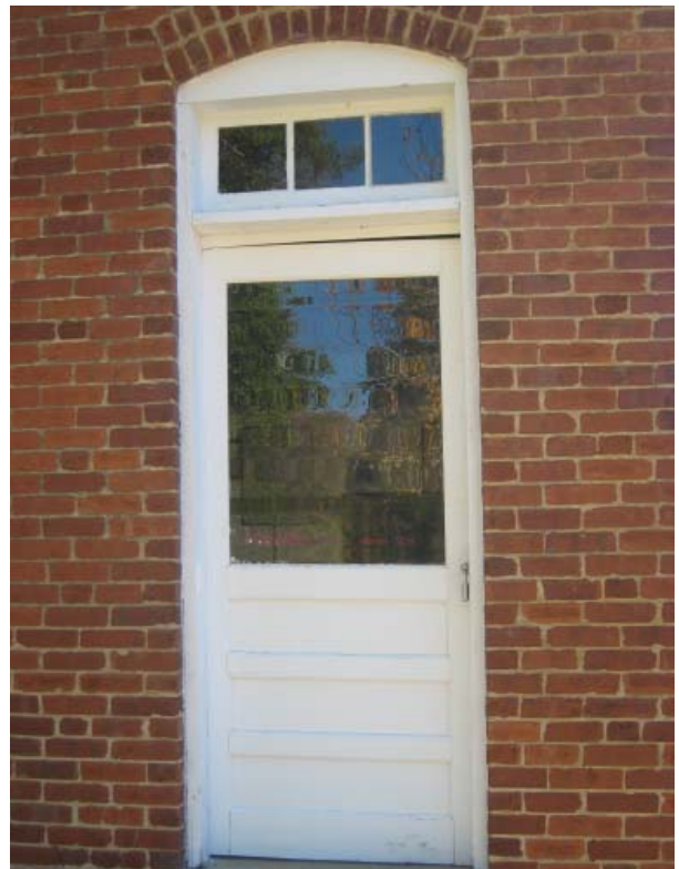
Figure 66. Original south doorway of west elevation.
