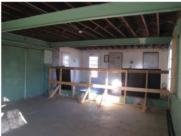
Figure 44. Northeast oblique view of first floor.
