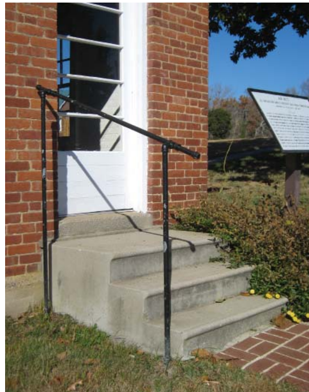
Figure 69. Pre-cast cement steps to east elevation doorway.
