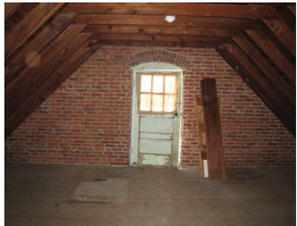
Figure 100. East gable wall.
