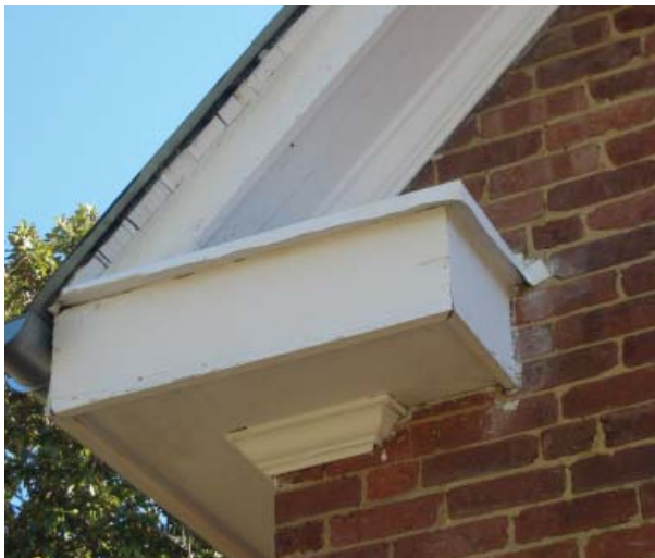
Figure 56. Roof cornice return.
