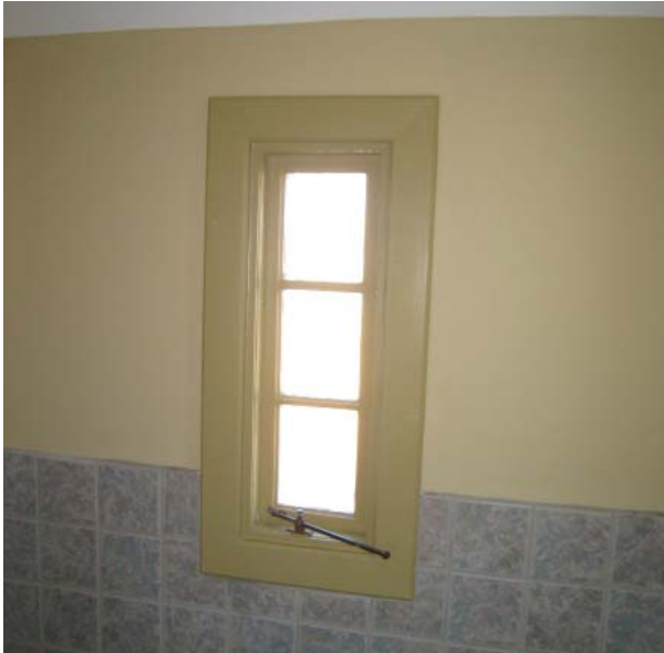
Figure 136. Typical casement window.
