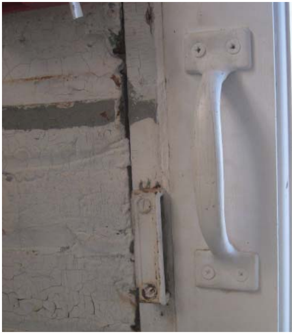
Figure 96. Original rimlock keeper and modern 5" handle of south door.
