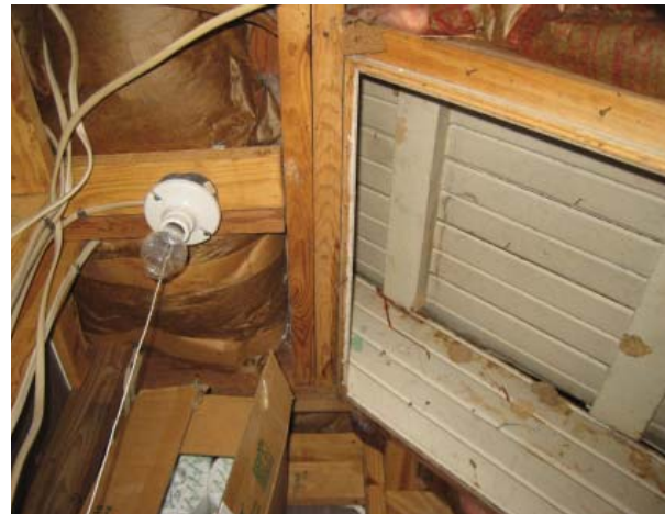
Figure 138. Access to roof hatch in Service Closet.
