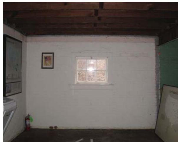
Figure 83. South wall of east section.
