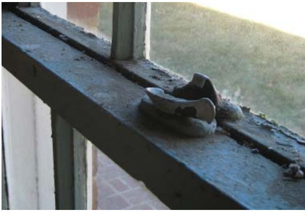
Figure 59. Typical latch for double-hung windows.
