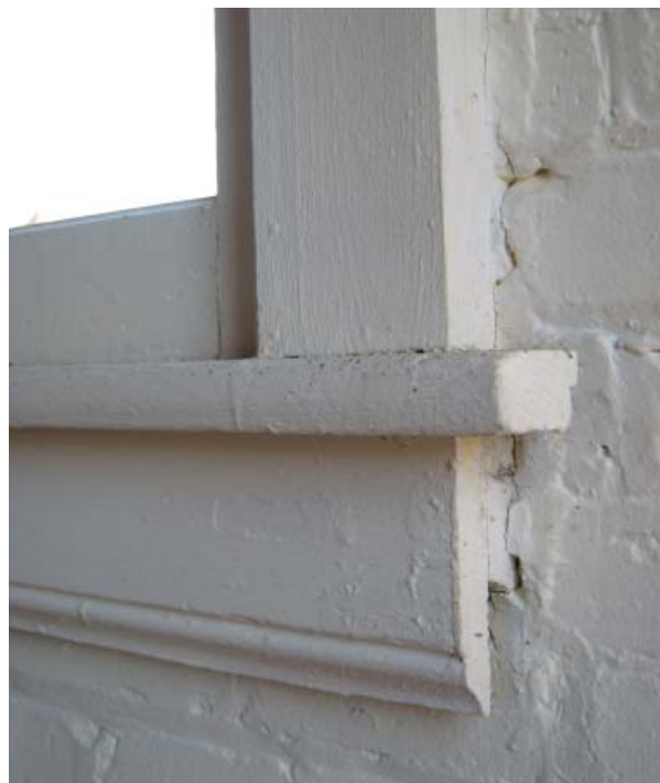
Figure 58. Typical window apron.
