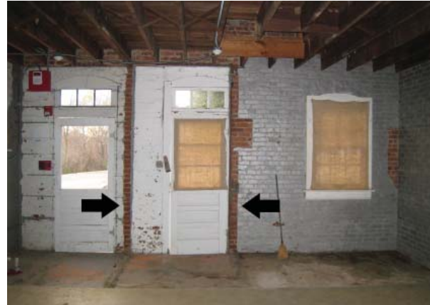
Figure 92. West wall of west section. Note imprints of partition walls added to enclose the restrooms.
