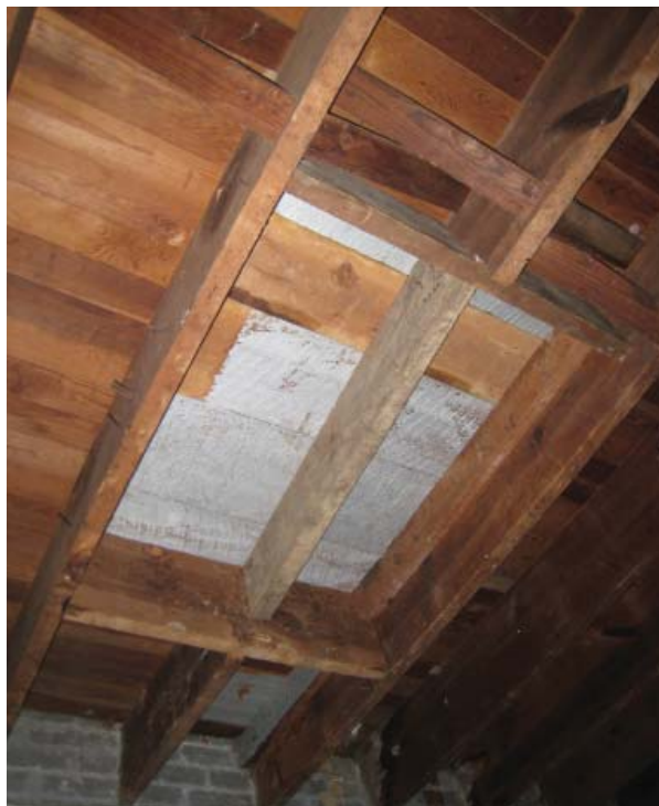
Figure 85. Hatch in ceiling was added.
