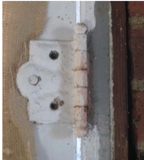
Figure 98. Clamshell door hinge on added center doorway.
