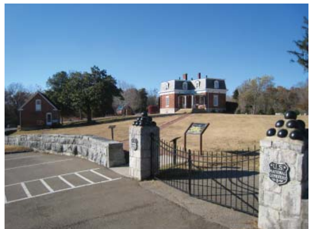
Figure 32. View of Carriage House/Stable, Pump House, and Lodge from cemetery grounds entrance gate with modern wheelchair/pedestrian entrance.
