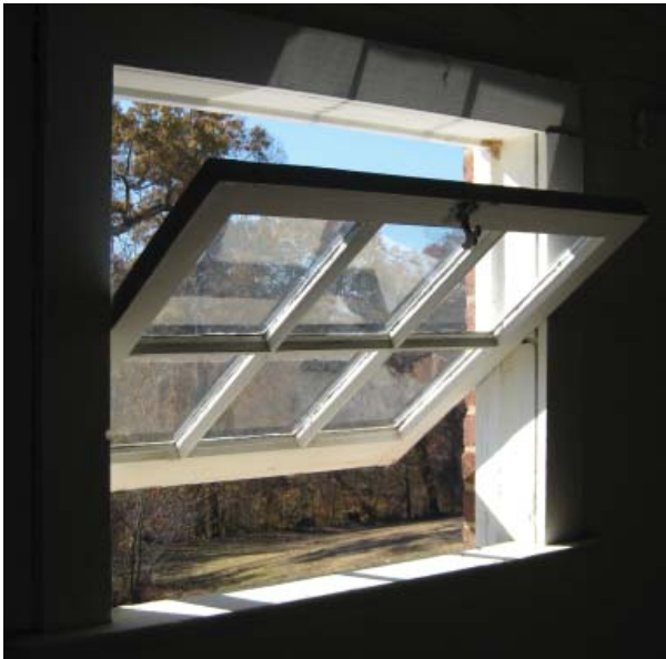
Figure 60. Pivot window, interior view.
