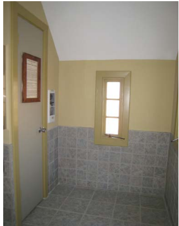
Figure 135. Alcove with doorway to Service Closet on north side of restroom.
