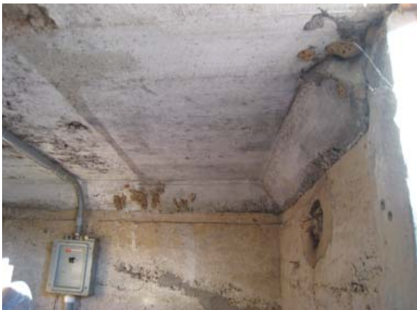
Figure 74. Added cement “cornice” visible on east and south walls.
