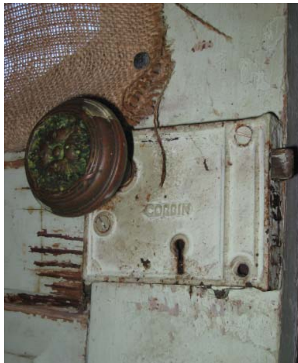
Figure 102. Original rimlock of east gable door.
