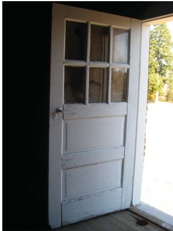
Figure 101. Original door, east gable.
