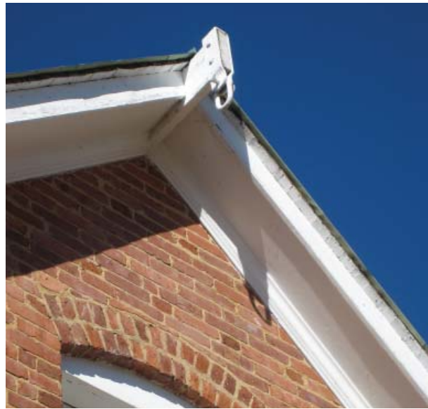
Figure 42. Hoist on end of extended ridge pole at east gable.
