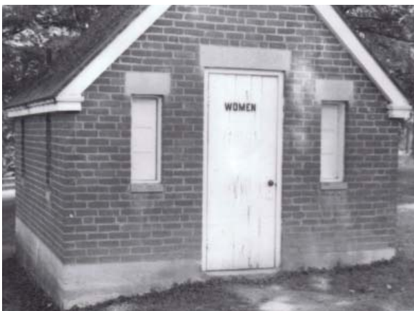
Figure 108. East gable end shown in 1964 shows cast stone sills and lintels, small walkway leading to door. (FODO collection)
