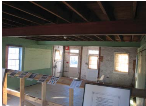
Figure 45. Southwest oblique view of first floor.
