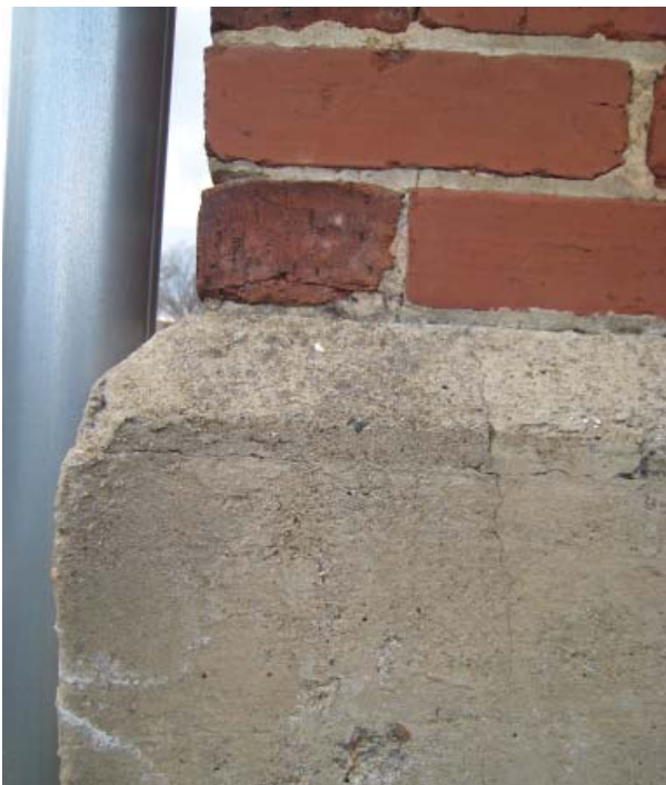
Figure 46. Concrete foundation with brick exterior walls.
