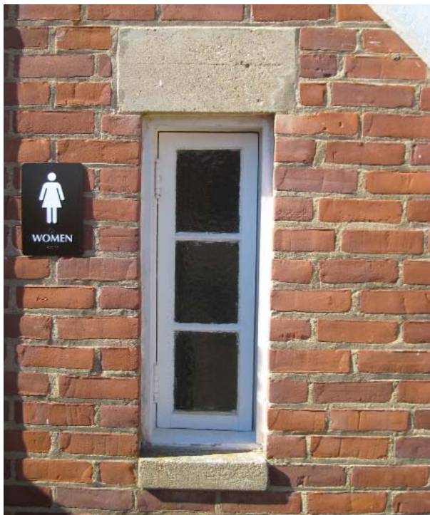
Figure 116. Cast stone sill and lintel.
