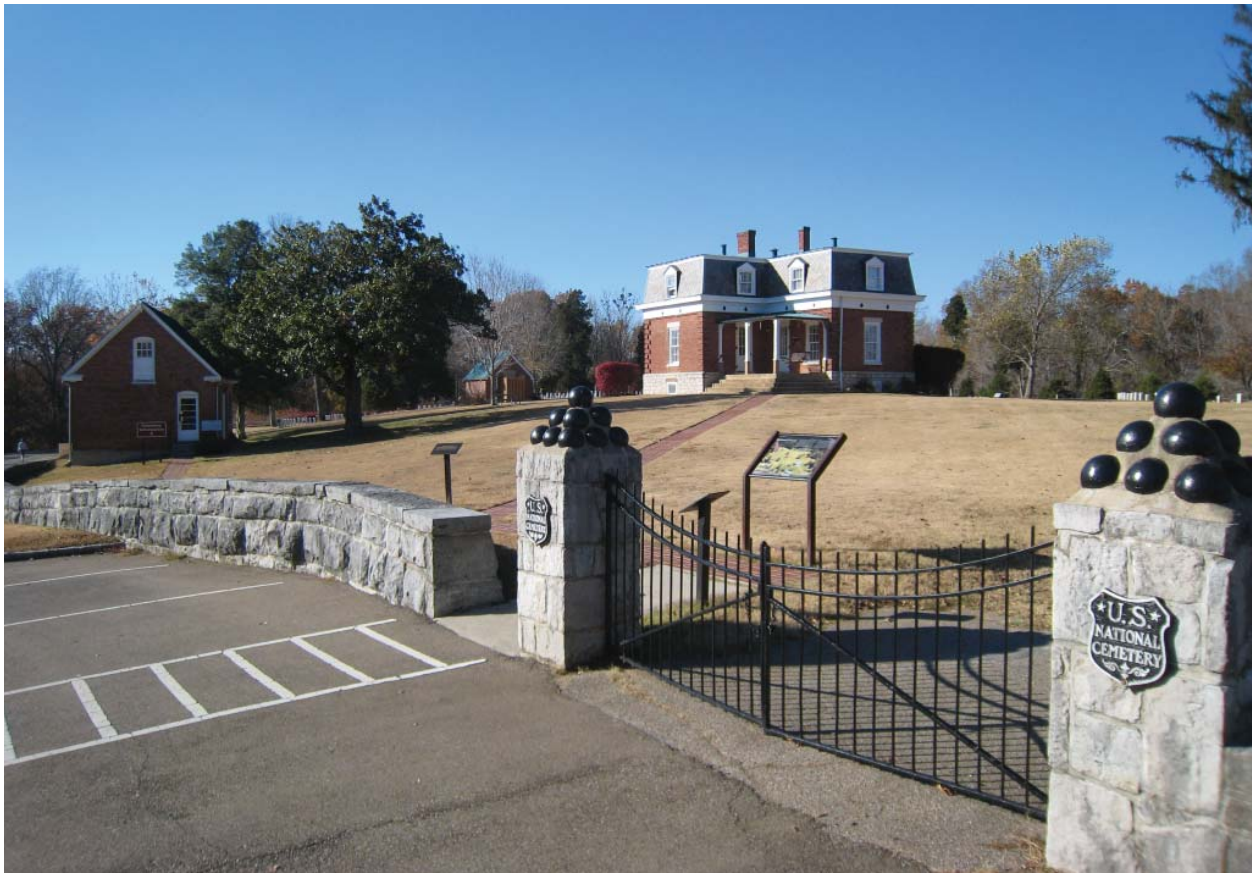
Figure 15. Entrance to National Cemetery showing Carriage House/Stable, Pump House, and Lodge, 2010.
