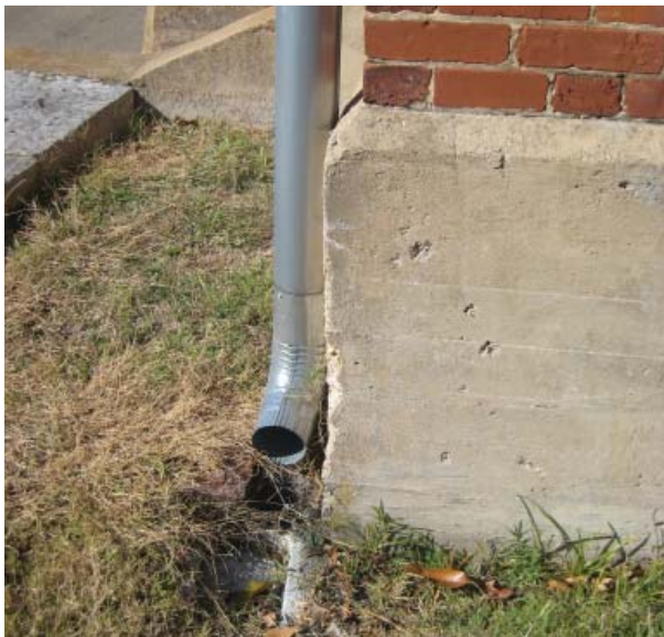
Figure 55. Downspouts dump rainwater at grade.
