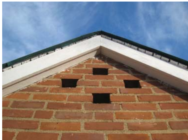
Figure 118. Pierced gables for ventilation.
