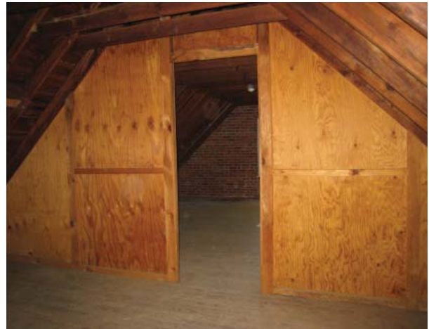
Figure 99. Added partition wall (west wall of Room 201).
