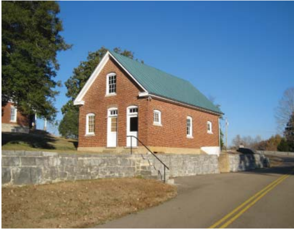
Figure 33. Southwest oblique view of the Carriage House/Stable as seen from the service road.
