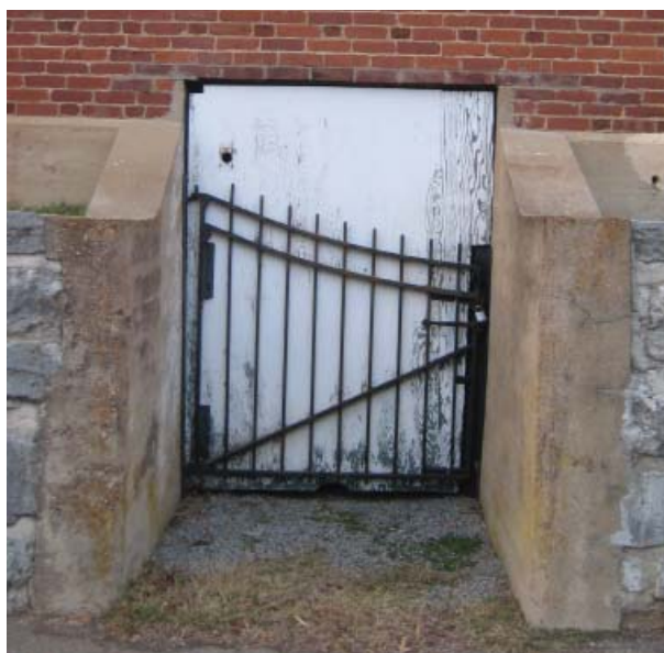
Figure 16. Basement entrance showing metal gate, 2010. (2010 photos were taken by the author.)
