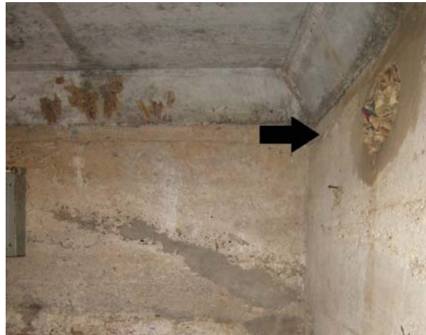
Figure 76. Opening for flue in south wall.
