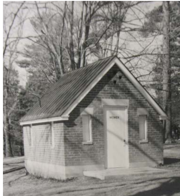
Figure 109. East gable end, ca. 1966, shows addition of concrete pad at entrance. (courtesy of Jaeger Company)
