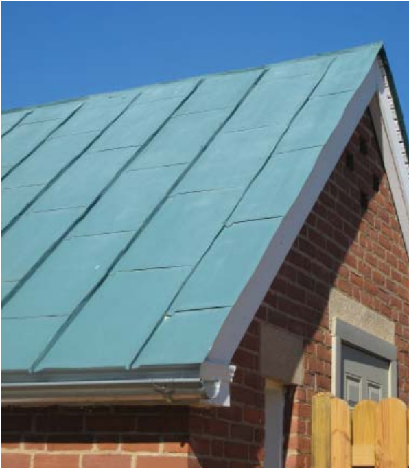
Figure 120. Standing-seam roof.
