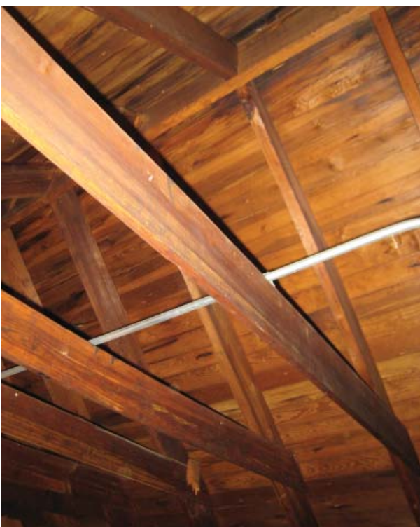
Figure 48. Collar beam at every pair of rafters.
