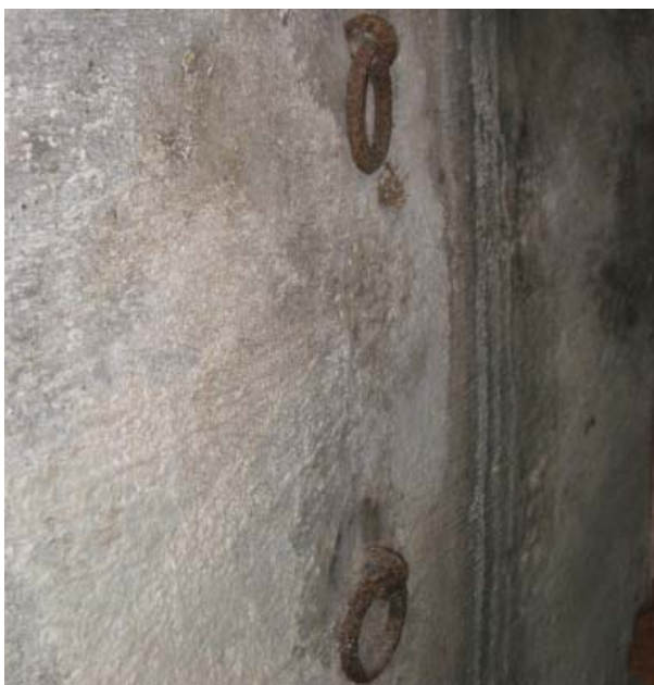
Figure 78. Two animal tie rings on west wall.
