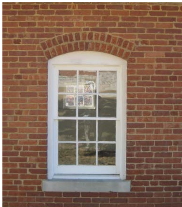
Figure 57. Typical double-hung sash window.
