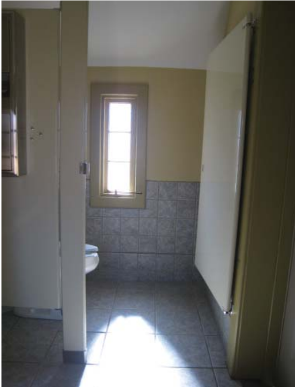
Figure 142. Toilet stall enclosure on south side of restroom.
