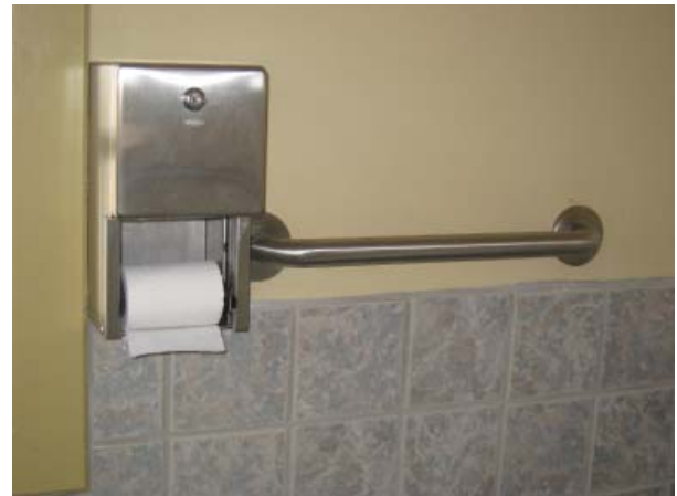
Figure 128. Typical grab bar and toilet paper dispenser.
