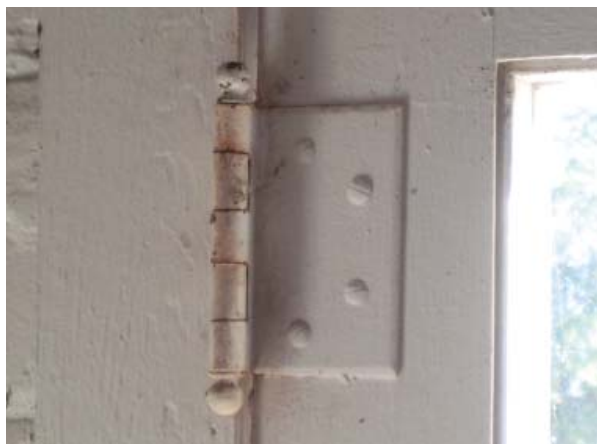
Figure 86. Original door hinges of first-floor east elevation door.
