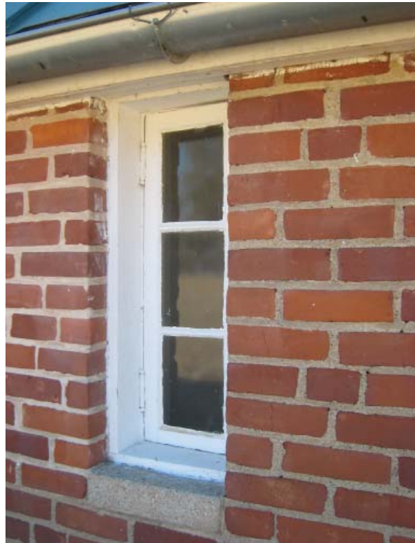
Figure 132. Typical casement window.
