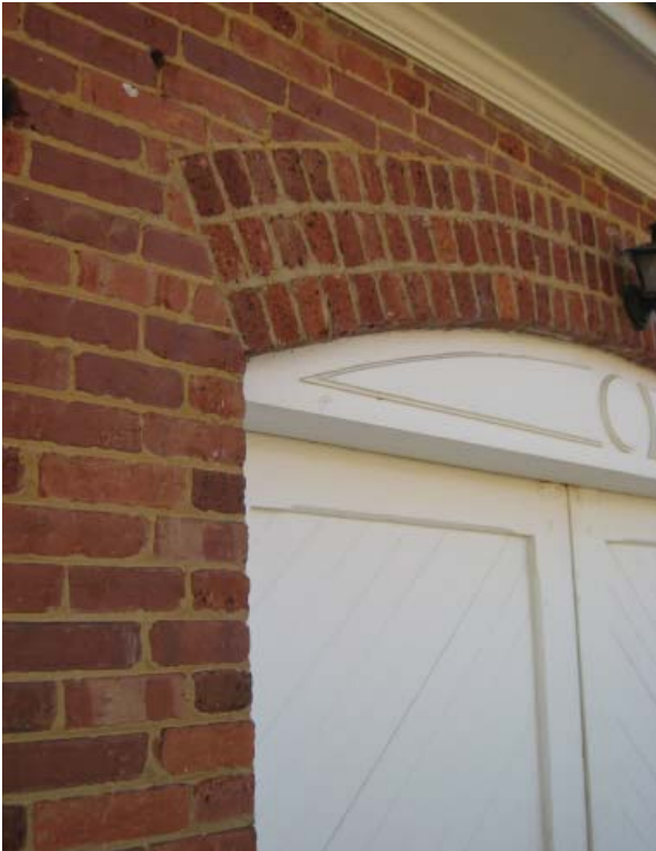
Figure 36. Dark brickwork with pattern of distressed brick headers.
