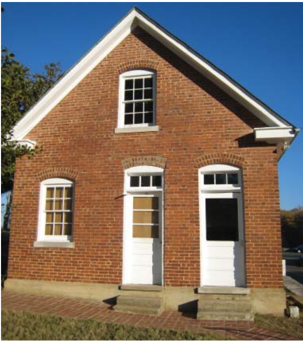
Figure 70. Two sets of concrete steps at west elevation.
