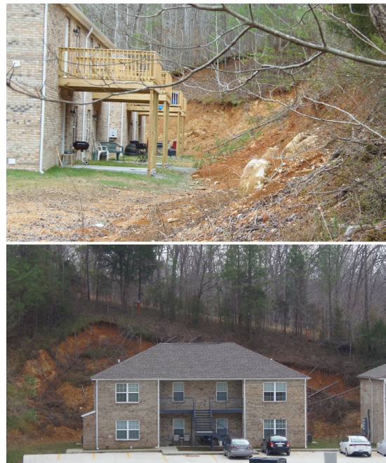
Figure 16. Photographs of a headscarp encroaching on the park boundary.
