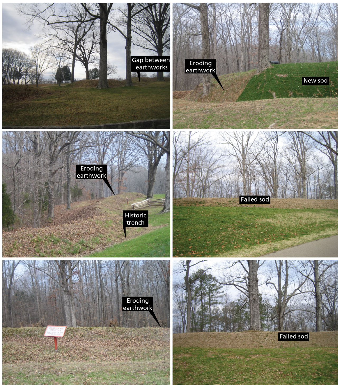
Figure 10. Photographs of eroding earthworks.
