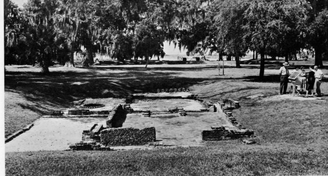
The families of Samuel Davidson and Dr. Thomas Hawkins lived side-by-side in this 18th century "duplex," the foundations of which were uncovered in archeological excavations of 1952.
