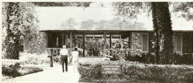
The new Fort Frederica Visitor Center constructed under Mission 66.
