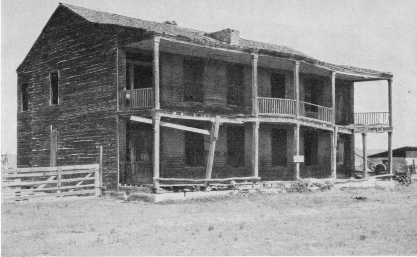
The building in 1938, prior to the commencement of restoration.
