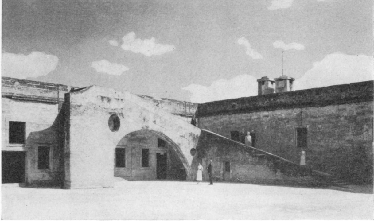
The stairway leading to the terreplein or roof of the fort was originally a smooth ramp up which the guns were dragged. The arch was rebuilt and the steps added about 1886. The iron bars in the windows were added by the Americans during the time the fort was used as a prison.
