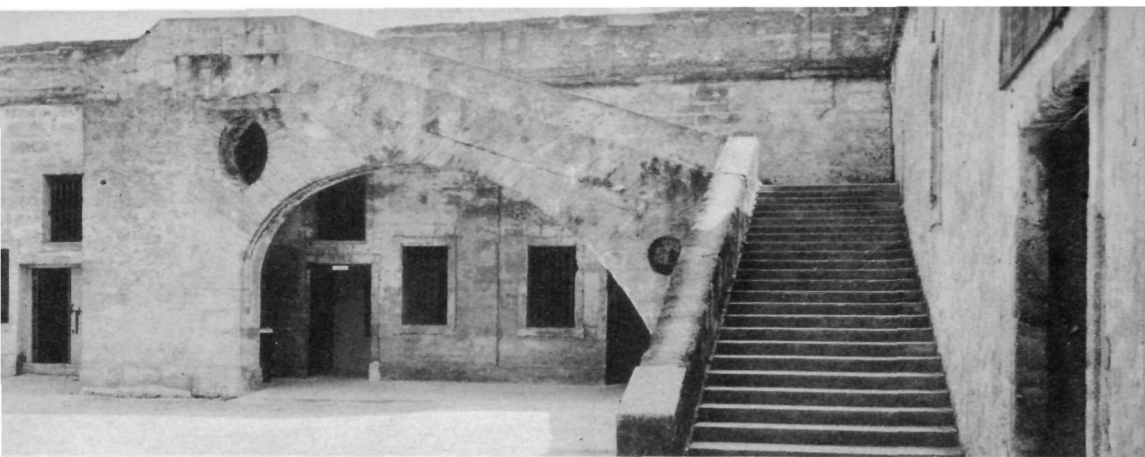
Arch Supports Ramp to Top of Fort Marion
