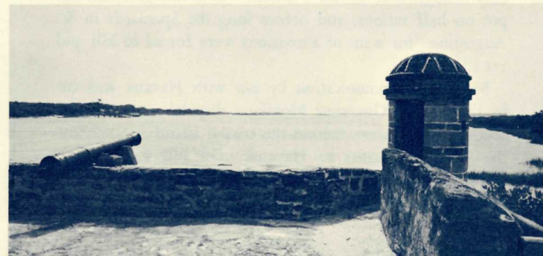
The tower commands the inlet.
