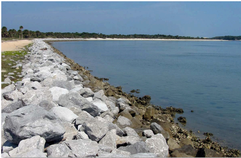
Figure 7. Revetment placed in 1977 to close the dike breach on Rattlesnake Island (#14 Figure 5). View is upriver (northwest) (image by Kate Dallas).
