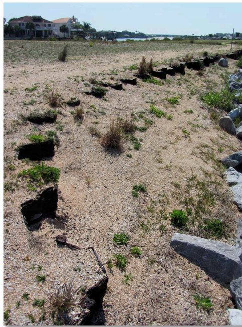
Figure 4. The top of the 1936 steel sheet pile dike buried in fill along the southwest shore of Rattlesnake Island (#17 Figure 5). View is to the southeast (image by Kate Dallas).
