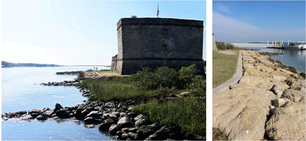
Figure 8. Groins, revetment, bulkhead, and ferry dock at Fort Matanzas in 2011 (#1–7 Figure 9). Left image looks downriver (southeast), while right image looks upriver (northwest) (images by Kate Dallas).
