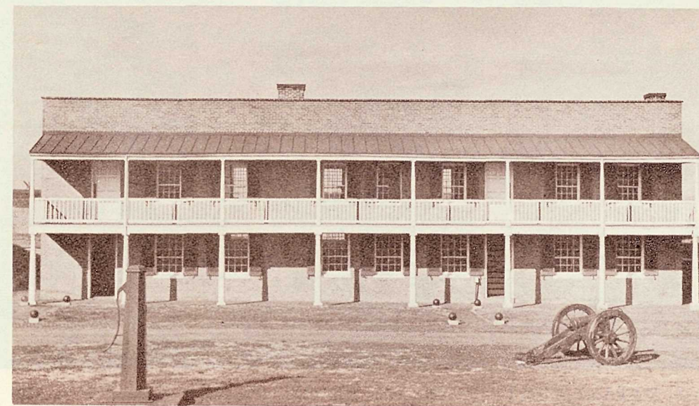
Old Barracks building, now used as a museum
