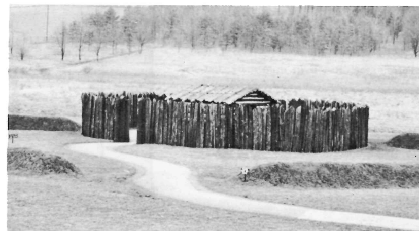
Reconstructed Fort Necessity.
