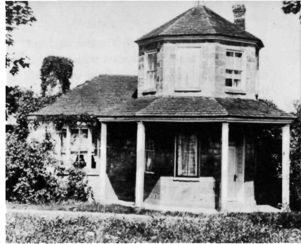
Old tollgate house built in 1814 on Old National Pike.
