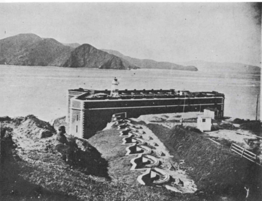
Fort Point, ca. 1869, showing cannon in place on the barbette ties. The sites of the 42-pound land batteries were obliterated during construction of the Golden Gate Bridge.
