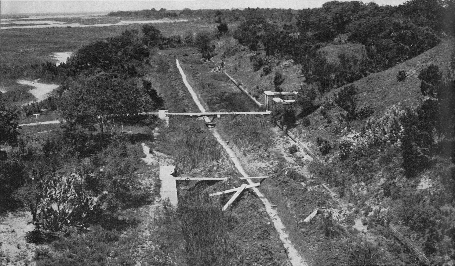
The demilune moat at Fort Pulaski before restoration.
